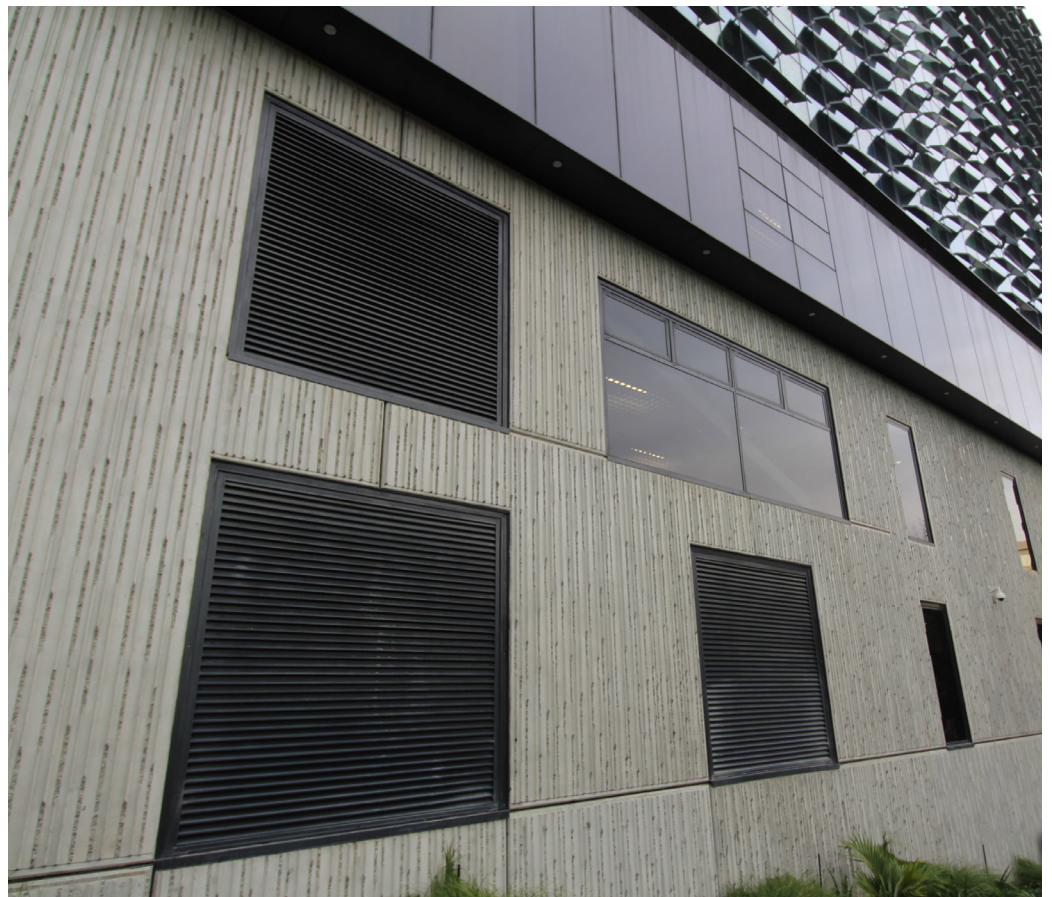
100mm Double Bank Mechanical Air Louvres integrated into curtainwall and rainscreen - University of Auckland, Engineering B405.
