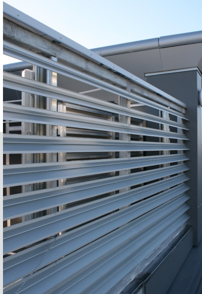
GHD Building NAPIER STREET, AUCKLAND
