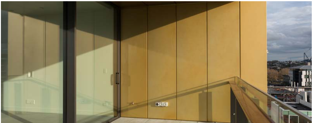
Halsey St, Auckland - RS1000 Cladding System
