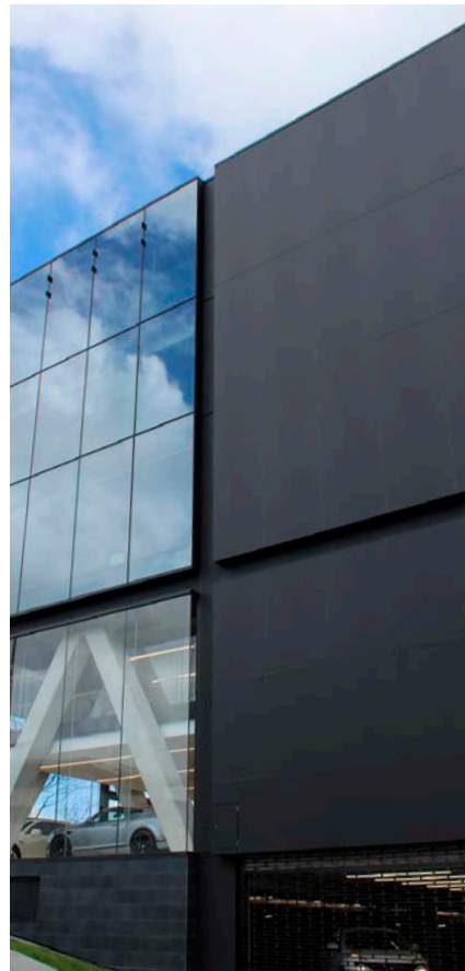
Giltrap Prestige Building, Auckland - WS1000
