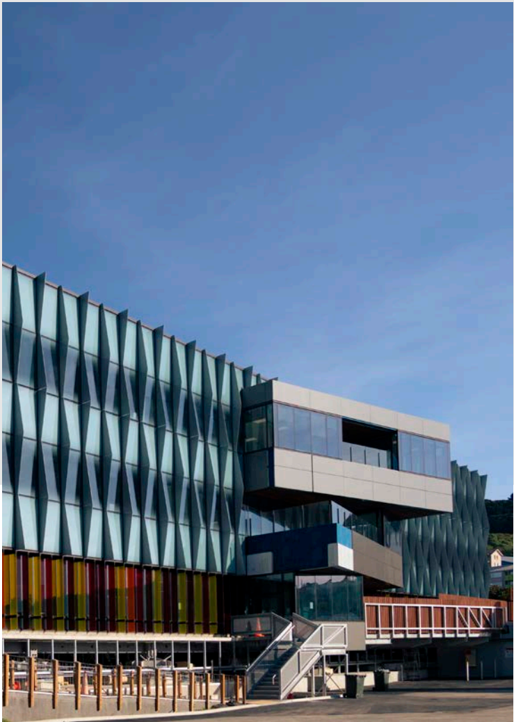
Wellington Regional Children's Hospital - RWS1000 cladding system
