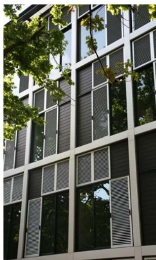
University of Auckland, Thomas Building - Integrated sunscreen louvre sliders.
