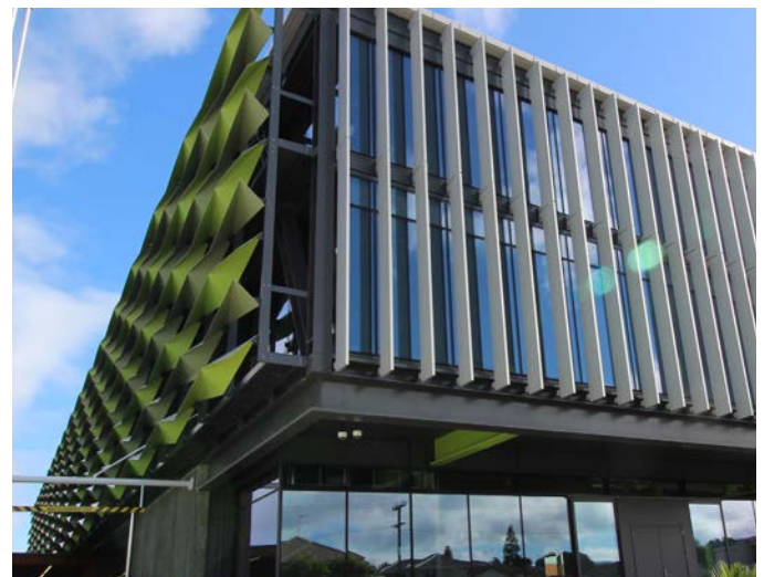
Zespri, Tauranga - Aluminium vertical fins and horizontal shading elements.
