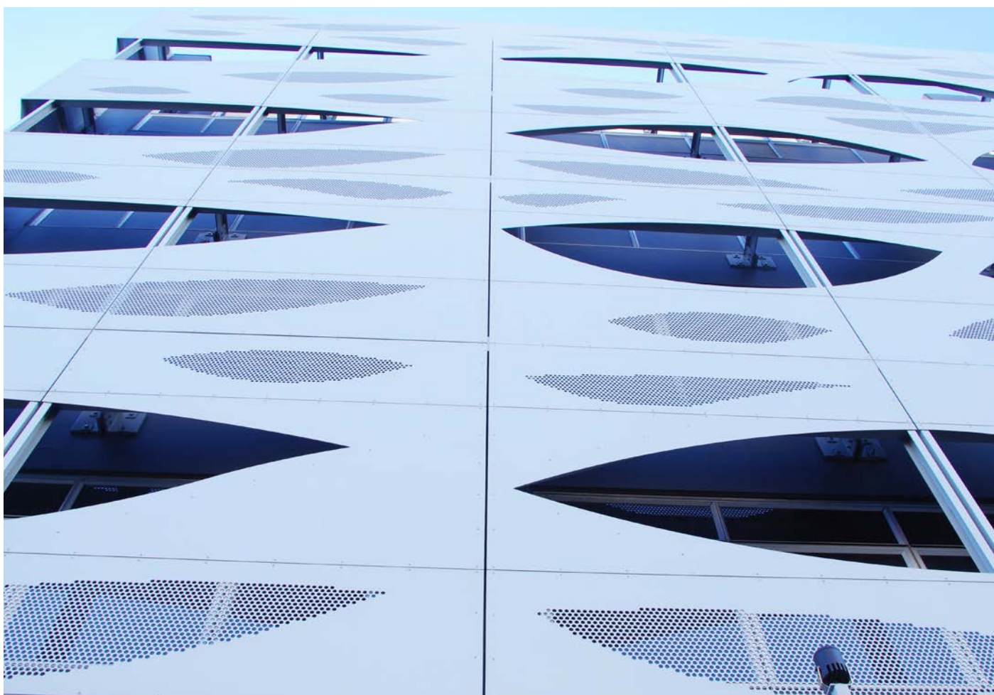
15 Huron Street, Takapuna, Auckland - Laser cut and perforated solid aluminium solar shade screens
