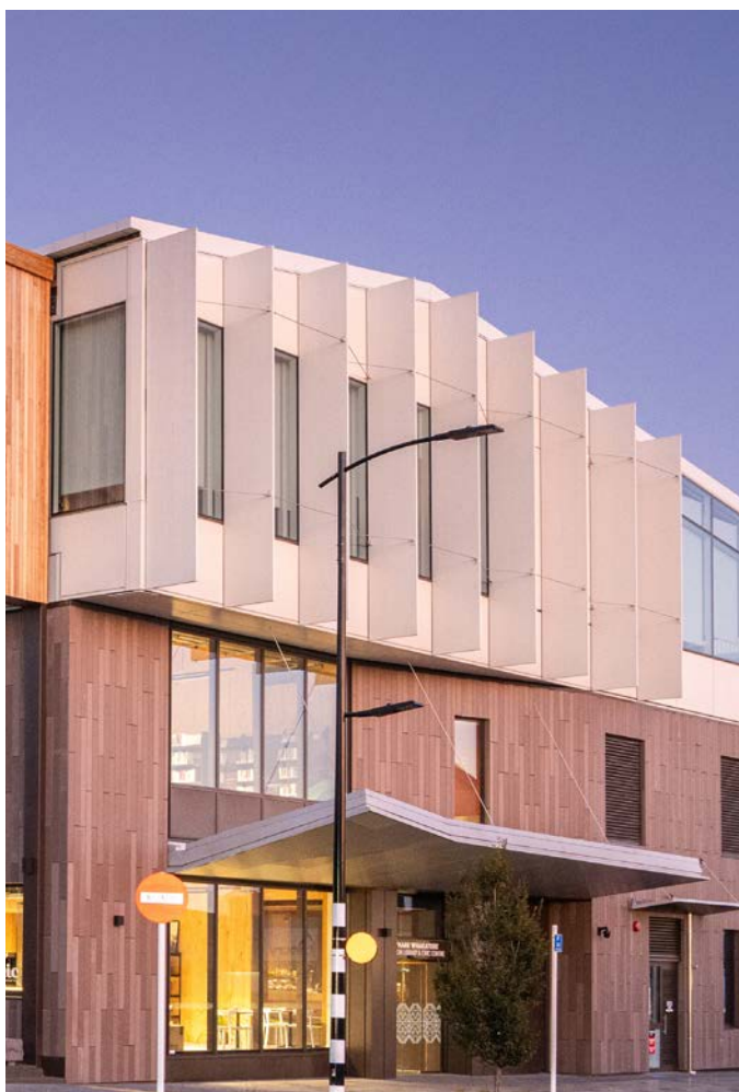
Ashburton Civic Centre & Library, Te Whare Whakere - Thermosash PW1000 unitised curtainwall integrated with vertical solar shading fins with actuators
