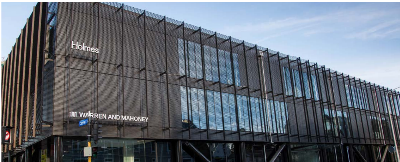
Warren & Mahoney offices in Christchurch - Shadegrate™ installed as solar shading to exterior facade.
