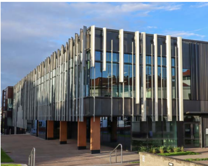
Massey University Innovation Complex - Extruded aluminium solar shading integrated into facade.
