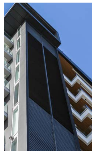
Oxford Terrace Apartments, Christchurch - Operable vertical elliptical louvres providing shading and privacy.
