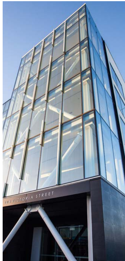
104 Victoria Str, Christchurch - PW400 Unitised Curtainwall with integrated vertical fins
