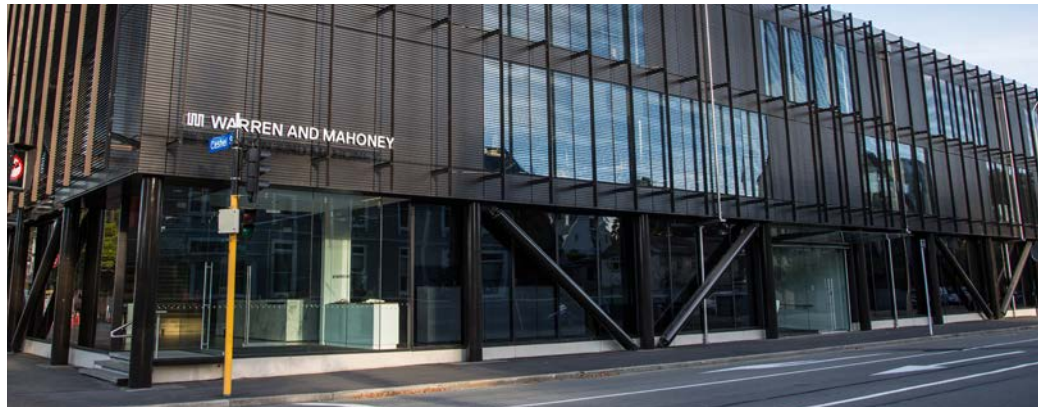
Warren and Mahoney Offices, Christchurch - PW400 Unitised Curtainwall with channel glazing & opening sashes to ground floor
