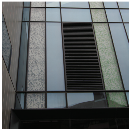
100mm Double Bank Mechanical Air Louvres integrated into curtainwall and rainscreen - University of Auckland, Engineering B405.
