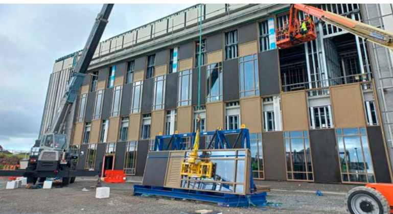
Latter Day Saints, Auckland site installation - PW1000 unitised curtainwall with integrated glazing, aluminium louvre and non-vision panel.
