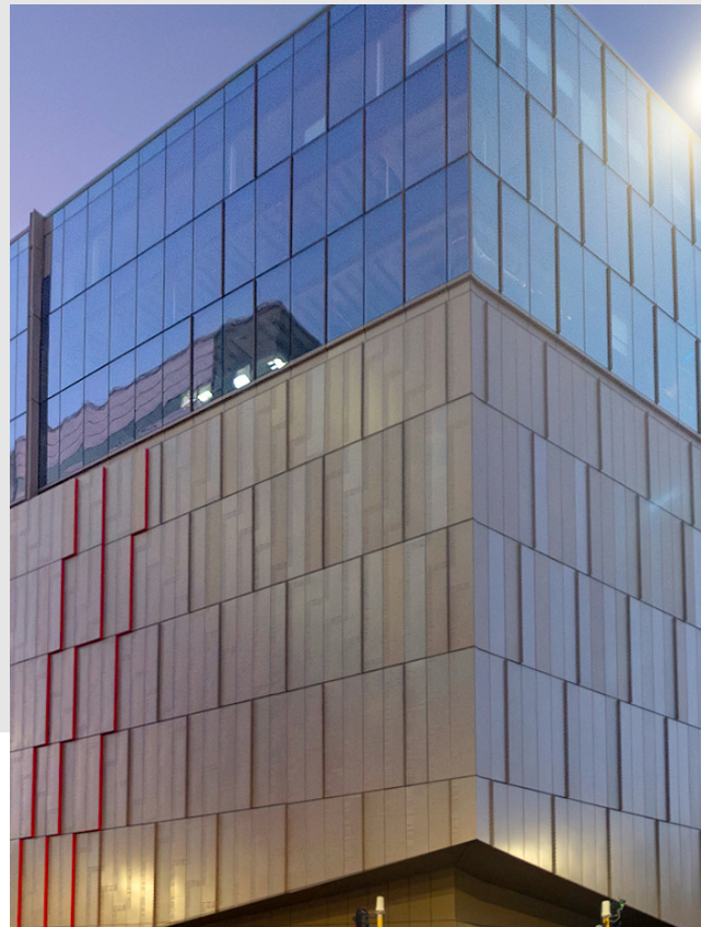
The National Archives Heke Rua building in Wellington - features a Thermosash PW1000 Thermally Broken unitised curtainwall compliant with BS/EU 16893 - a factor of 10 better air infiltration / ex-filtration than NZS4284 compliance.
