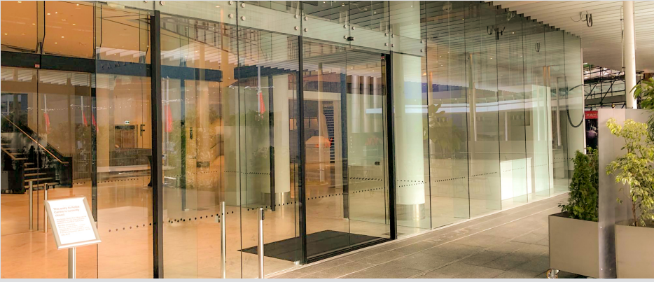
Aotea Events Centre, Auckland CBD - channel glazed atrium incorporating glass auto doors
