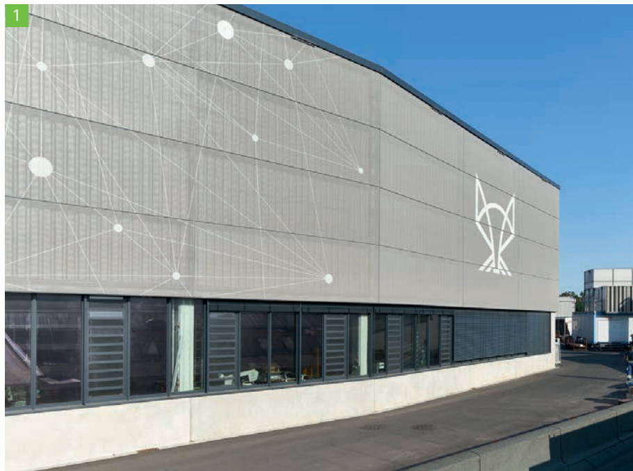
Otto Fuchs KG office building, Meinerzhagen
