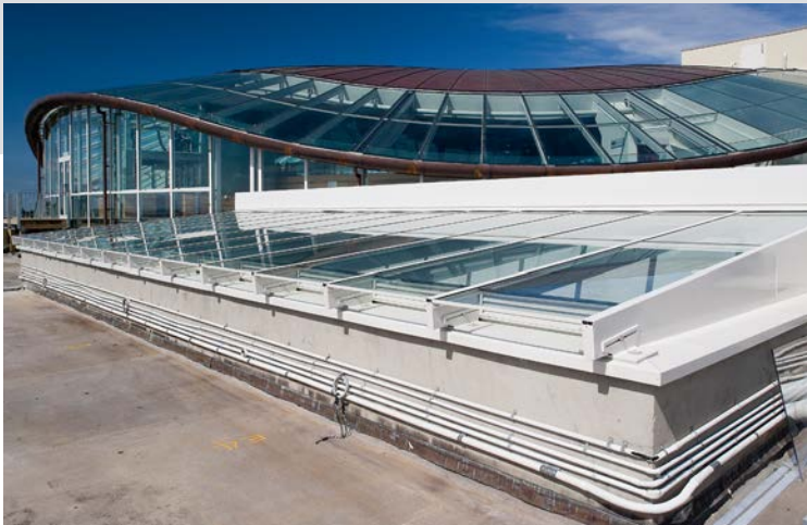
Auckland Museum "The Dome" and rooflights
