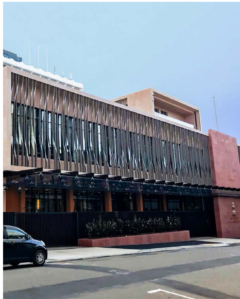
High Commission of India, Wellington - featuring Thermosash PW1000 unitised curtainwall with integrated sliding doors, ballistic rated windows, and skylights.
