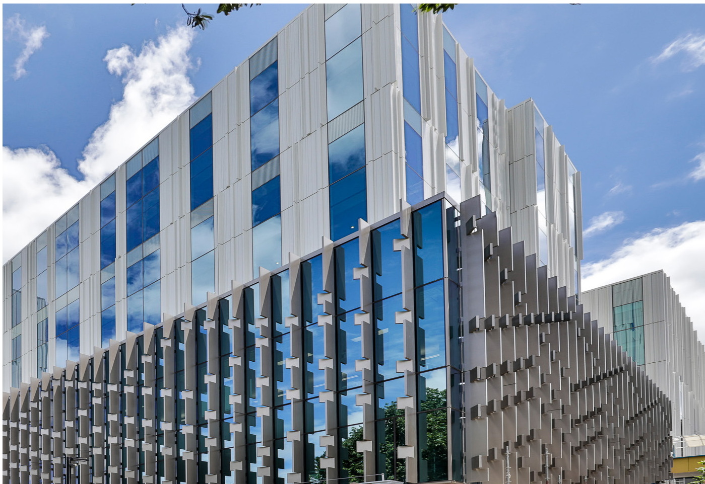
University of Auckland, B201 - Vertical solar shade feature fins integrated into PW1000 unitised curtainwall.
