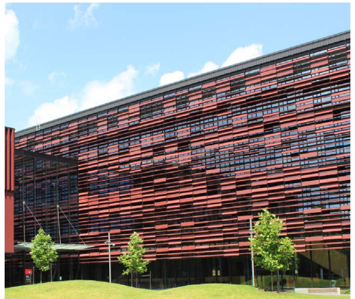
AUT M1, Mana Hauora Building - solar shading cantilevered off the PW1000 unitised curtainwall with a maintenance walkway incorporated behind the screens.
