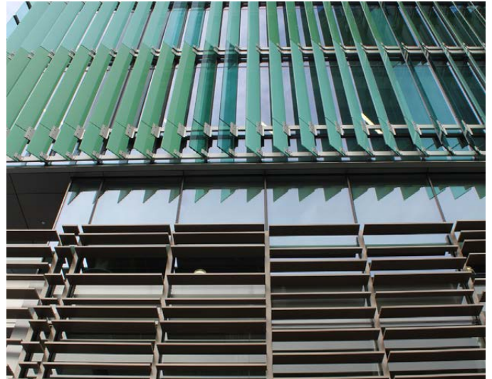
Fonterra Building, Fanshawe Street, Auckland - vertical and horizontal solar shading louvres
