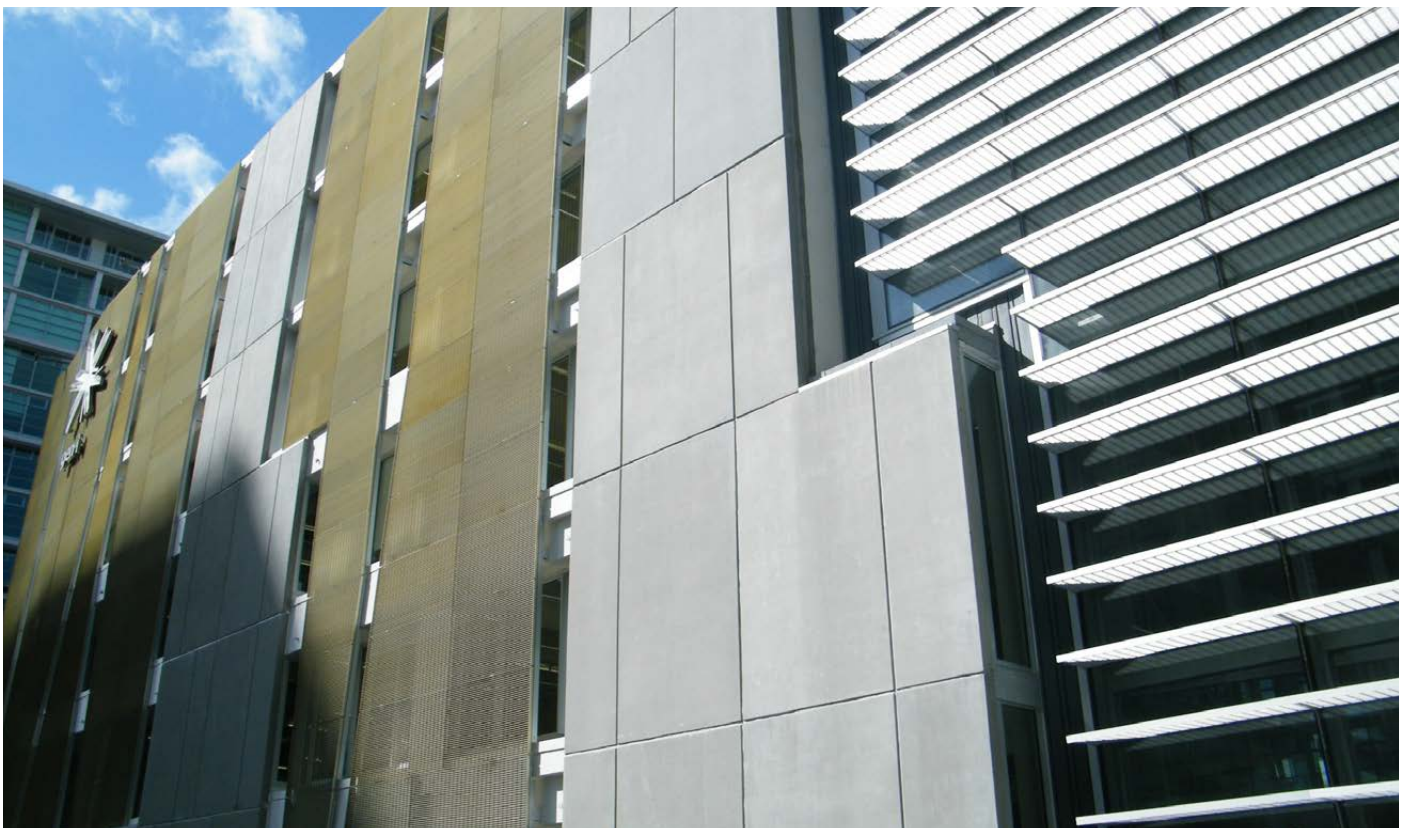
Telecom Willis Tower, Wellington - shadegrade™ and Shadetread™ installed as vertical and horizontal solar shading.
