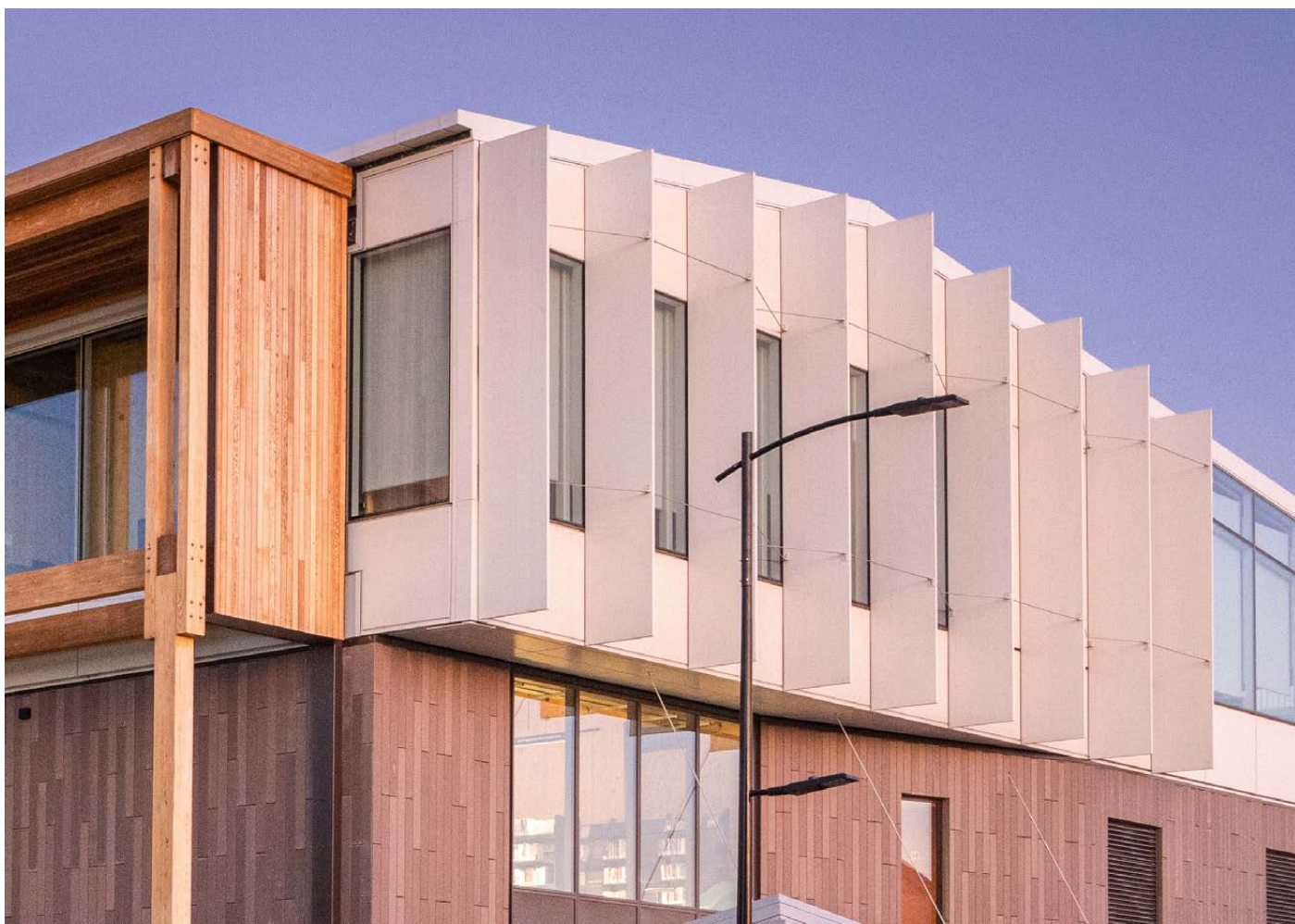
Ashburton Civic Centre & Library, Te Whare Whakere - PW1000 unitised curtainwall integrated with vertical solar shading fins with actuators
