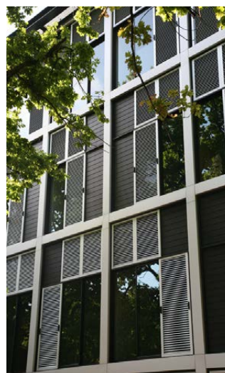
University of Auckland, Thomas Building - integrated sunscreens
