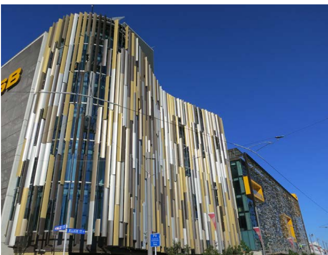
ASB North Wharf, Auckland - vertical solar shade fins suspended off the curtainwall.
