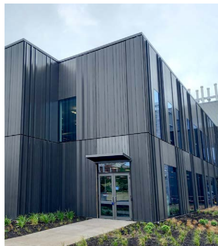
Massey Innovation Complex, Auckland - unitised extruded aluminium plank integrated with PW1000 HP Unitised Curtainwall.
