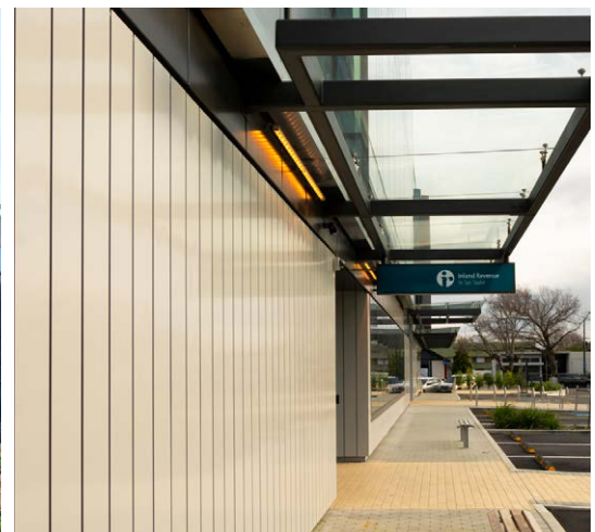
Te Ao Nui Building (IL4), Palmerston North - extruded aluminium plank vertical cladding.
