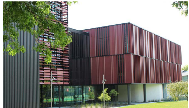
AUT M1 Mana Hauora Building - unitised aluminium planking provided a lightweight alternative to terracotta due to the floor spans on this project.
