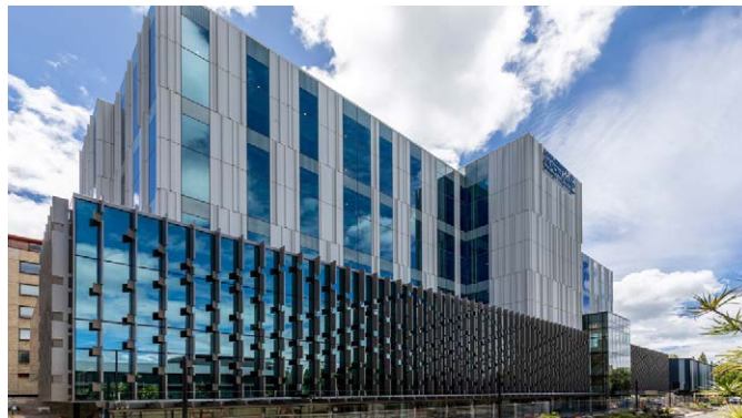
University of Auckland B201 - unitised aluminium planking integrated with PW1000 HP Unitised Curtainwall delivers an energy efficient envelope.
