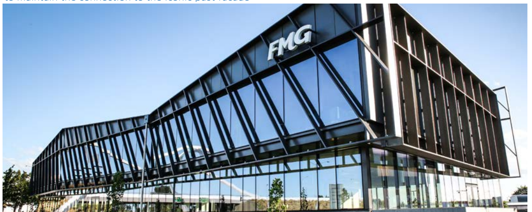
FMG Building situated at Christchurch Airport - PW1000 integrated with custom feature fins
