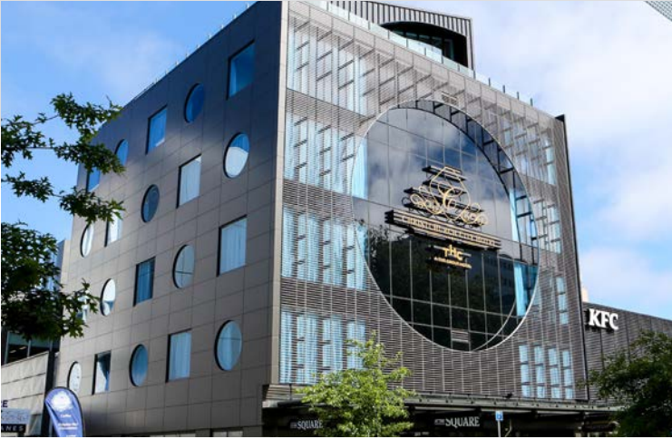
699 Comobo St Hotel, CHCH - PW1000 integrated with a custom solar shade
