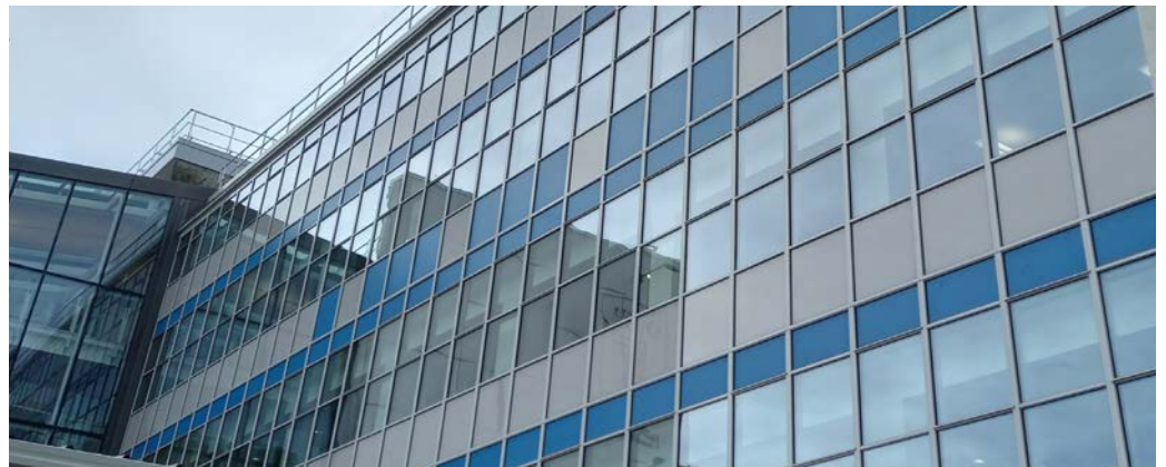
UOO Dental School, Walsh Building - PW1000 replicating the pattern and colour of the original 1960s design to maintain the connection to the iconic past facade
