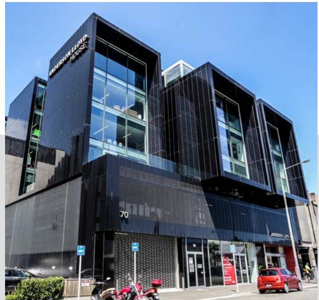
Anderson Lloyd House, Gloucester Str. CHRISTCHURCH - RS1000 SYSTEM
