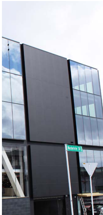
Giltrap Prestige Building, Auckland - WS1000
