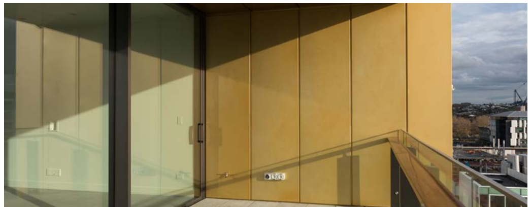
Halsey St, Auckland - RS1000 Cladding System
