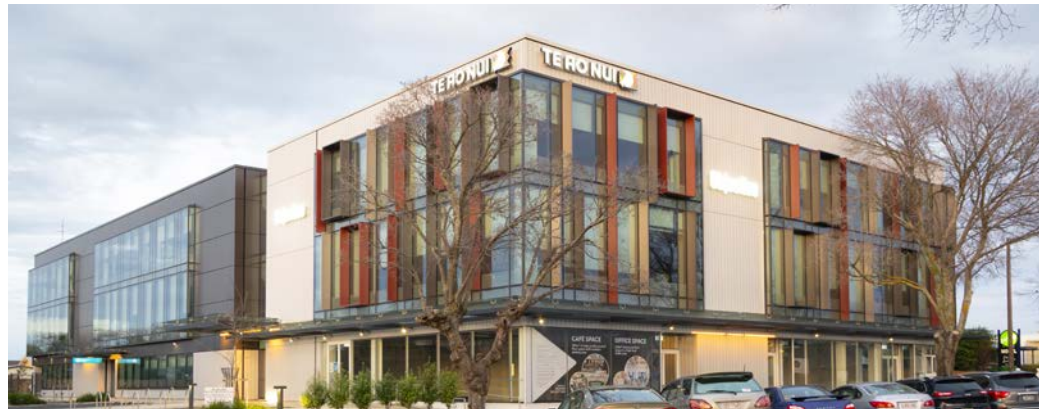
Te Ao Nui (IL4) Building, Palmerston North - RS1000 Cladding System hooked-on folded sheet metal and aluminium plank cladding, vertically and horizontally fixed.
