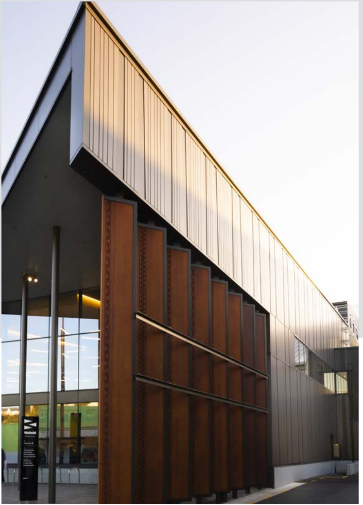
Johnsonville Library - RS1000 Cladding System incorporating powdercoated aluminium vertically and horizontally fixed
