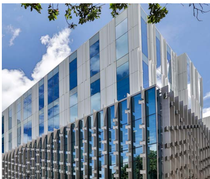
University of Auckland B201 - PW1000 unitised curtainwall integrated with vertical solar shading, and to upper level with Thermoplank.
