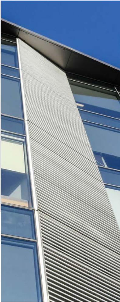
123 Victoria Street, Christchurch - PW1000 structural curtainwall integrated with horizontal aluminium louvres
