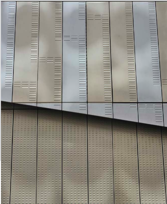
Detail of the prefabricated unitised embossed aluminium panels installed on National Archives Heke Rua, Wellington.
