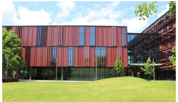
AUT M1 Mana Hauora Building - unitised aluminium plank provided a lightweight alternative to terracotta due to the floor spans on this project.
