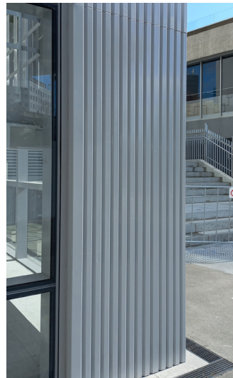
CAB Apartments, Auckland - unique folded metal cladding designed to match the original heritage fluting.
