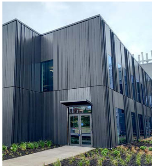
Massey Innovation Complex, Auckland - unitised extruded aluminium plank integrated with high performance curtainwall.
