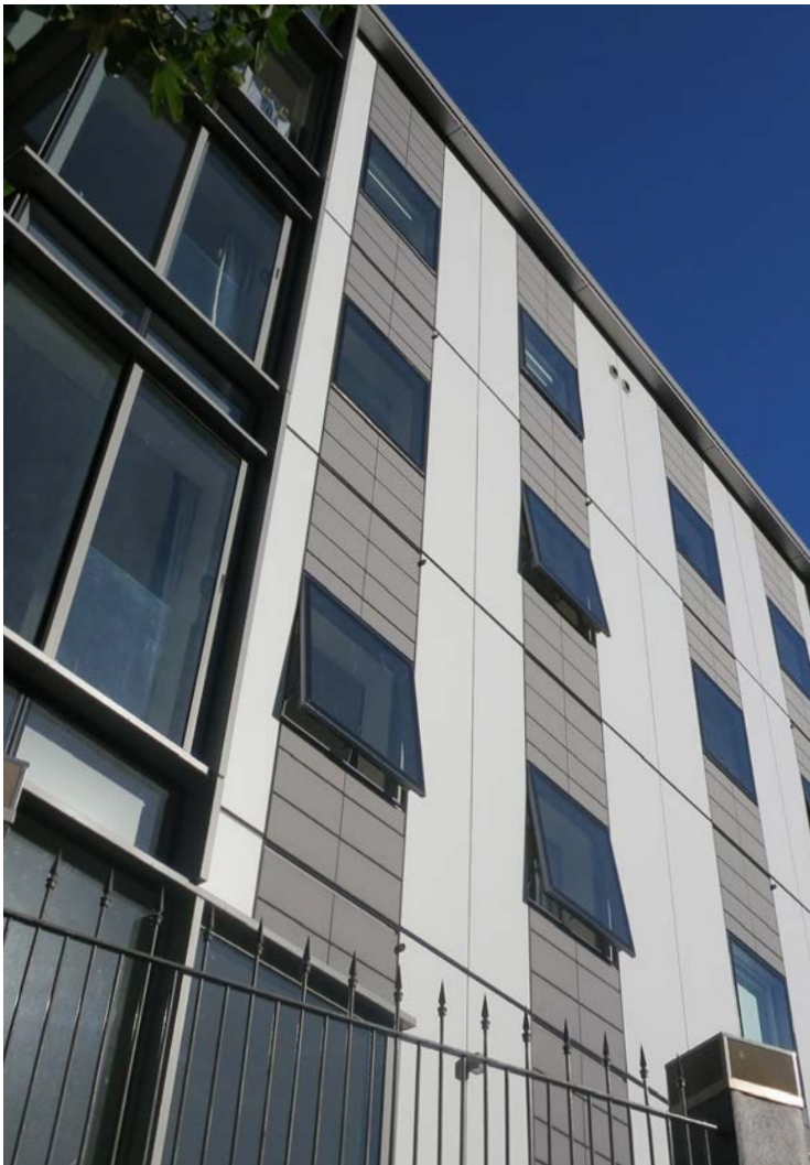
Columbia Apartments, Auckland - re-clad project which included flat solid aluminium panels powdercoated to compliment the integrated terracotta tiles.
