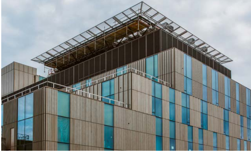
Taranaki Base Hospital East Wing, NEWB - features a variety of profiled unitised aluminium planking integrated into PW1000 high performance unitised curtainwall.
