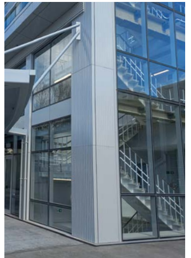
CAB Apartments, Auckland - unique folded metal cladding designed to match the original heritage fluting.
