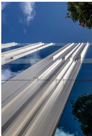
University of Auckland B201 - unitised aluminium plank profile.
