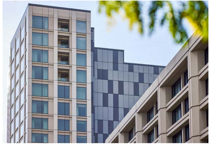
New addition to the Cordis Hotel, Auckland - flat solid aluminium panels with embossed powdercoating to maintain a look similar to the precast panel facade of the original hotel.
