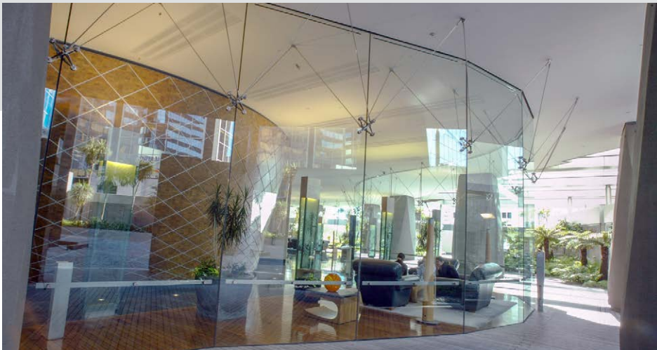
Royal Sun Alliance, Auckland - light weight structural tension cables and support fixtures on straight and angled channel glazing, provides minimal intrusive wind bracing
