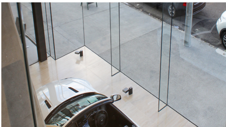
Channel glazing with integrated glass fins
