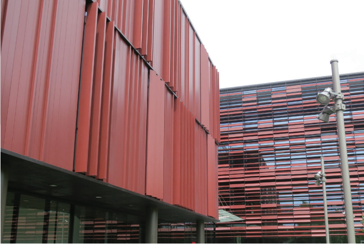
AUT M1 The Mana Hauora Building - facade planking (left), and horizontal solar shading cantilevered off unitised curtainwall
