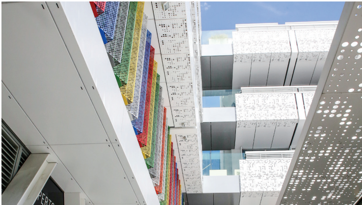
BNZ Cashel stage 2, Christchurch - perforated decorative sheet metal canopies and solar shading
