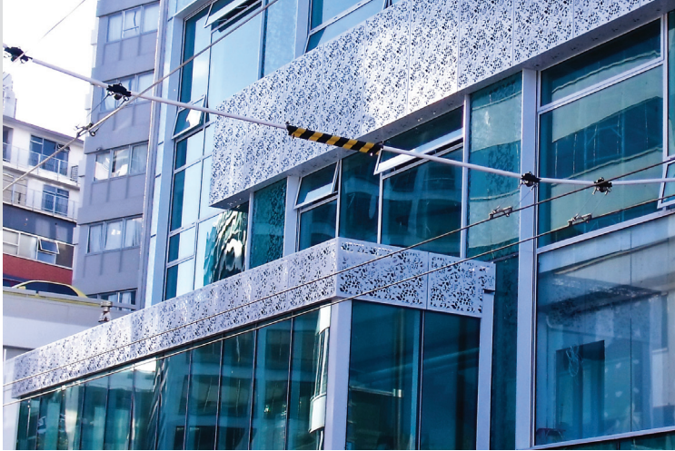
Regent Centre, Wellington - patternated perforated sheet metal balconies
