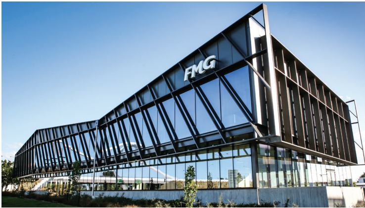
FMG Building - Christchurch - horizontal & diagonal fins with a complex T-section steel bracketry system to connect fins into curtainwall
