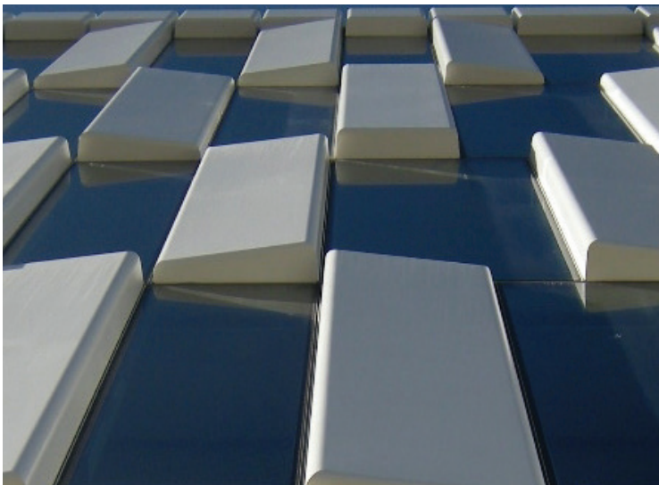
BNZ Harbour Quays, Wellington - folded metal pressings hung off curtainwall
