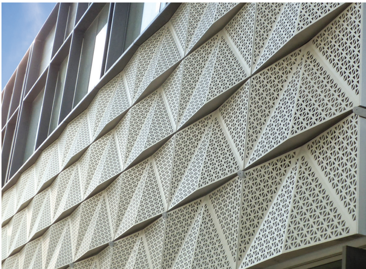
Bnz Cashel stage 1 - perforated and folded sheet metal installed as car park screening
