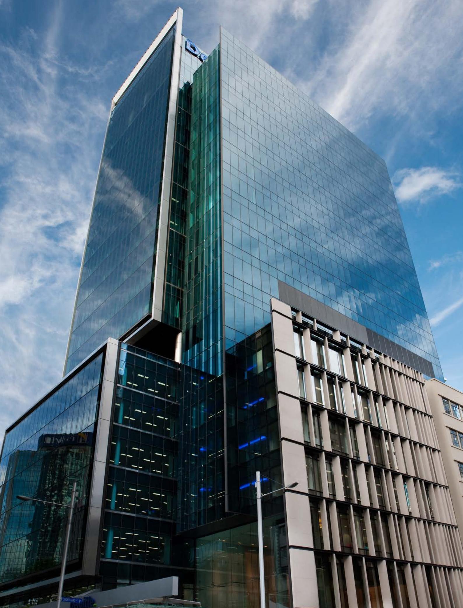
The twin skin high performance Thermosash PW1000 Unitised Curtainwall with low 'E' glazing maximises views and light whilst delivering passive ventilation.
