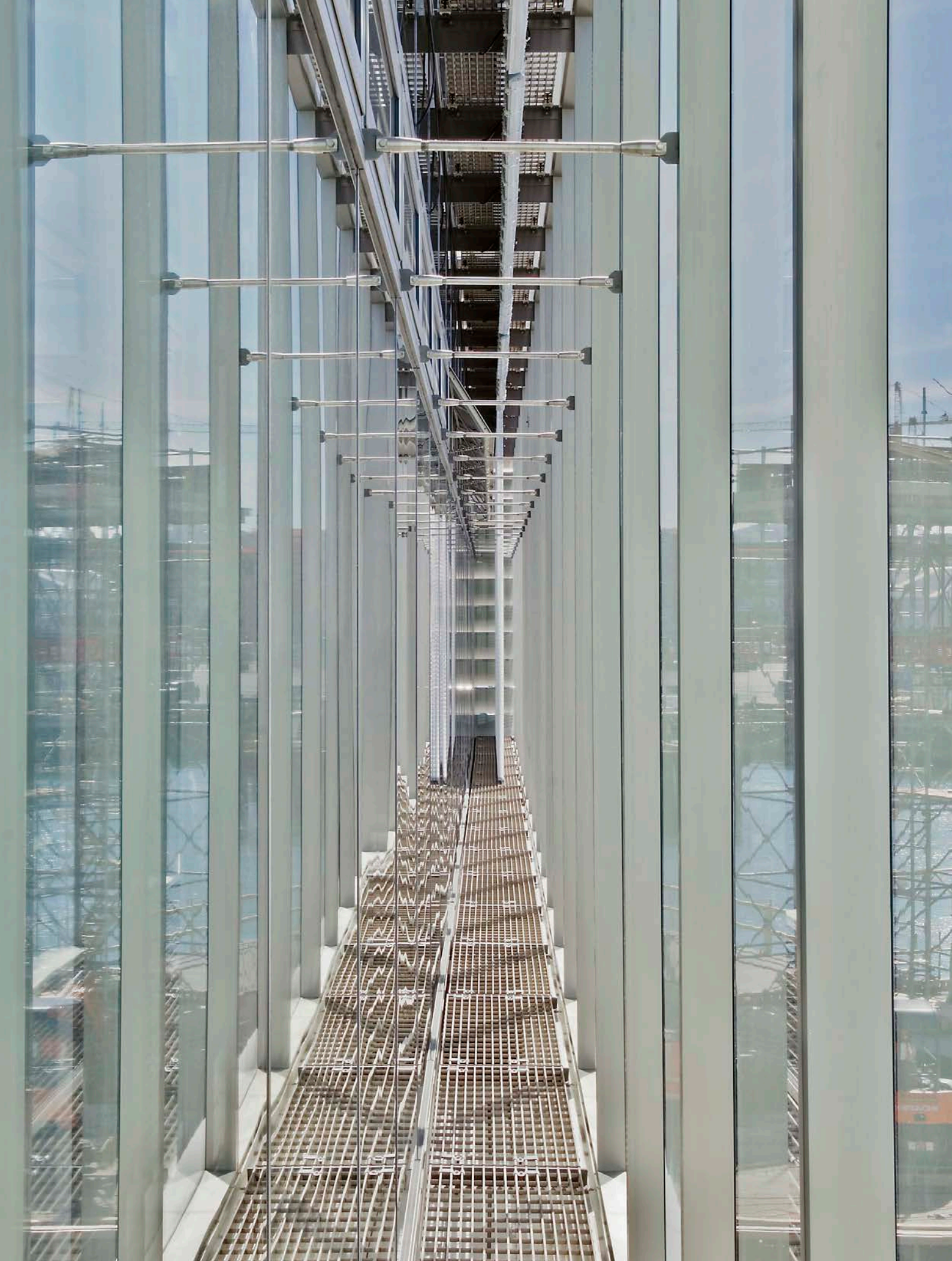
Meridian's high performance twin skin Thermosash PW1000 Unitised Curtainwall of anodised aluminium and transparent glazing integrated with maintenance walkways within the 400mm cavity.
