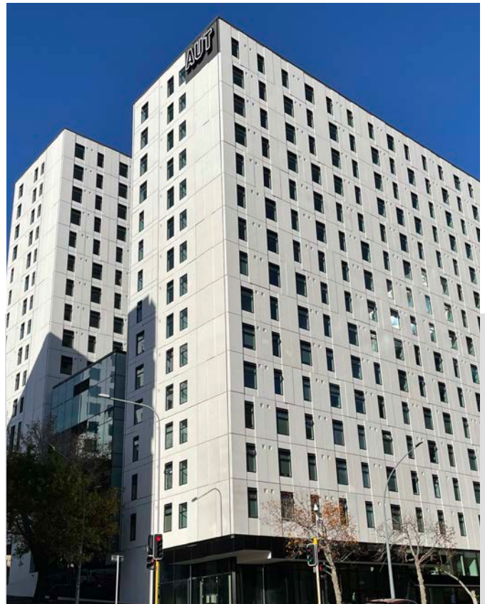
AUT Student Accommodation DELTA SUITE WINDOWS
