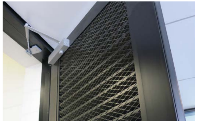
Door with MAL 40mm Single Bank and integrated vermin guard - St Cuthberts School, Centennial Pool Complex, Auckland.
