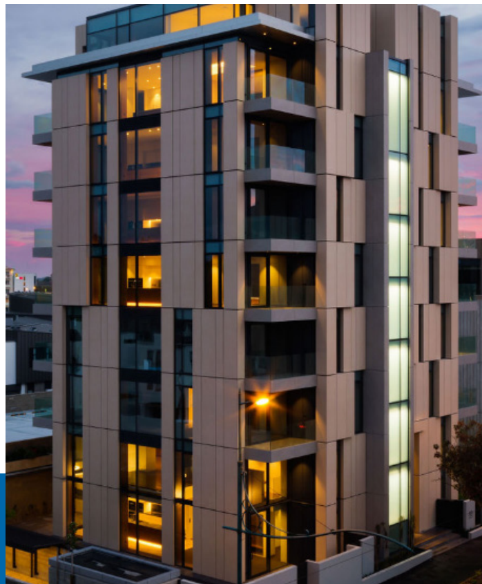
Paragon Apartments, CHCH - PW1000 integrated with large format porcelain
