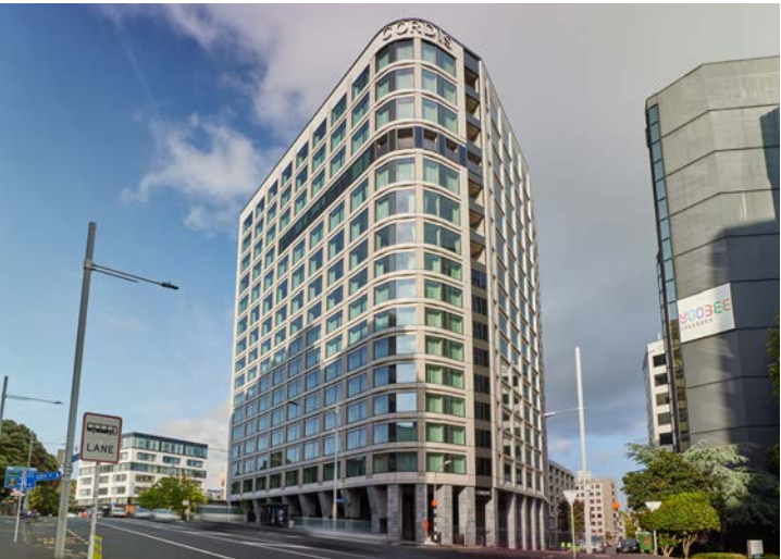
Cordis Hotel, Auckland - PW1000 Unitised Structurally Glazed Curtainwall
