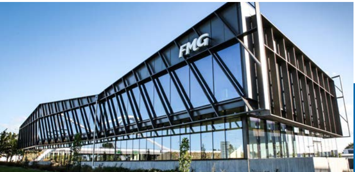
FMG Building situated at Christchurch Airport - PW1000 integrated with custom feature fins.
