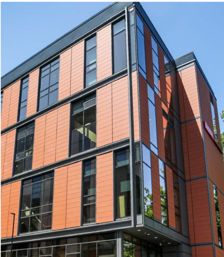
UOC Beatrice Tinsley Building - PW1000 integrated with terracotta tiles
