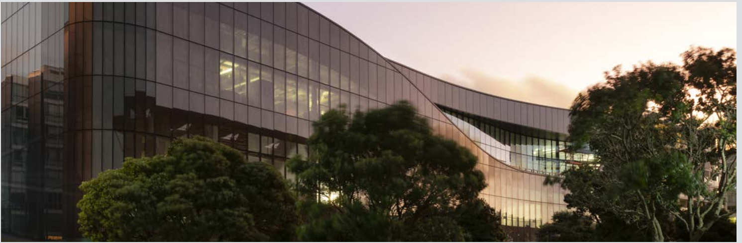
Tākina Wellington Convention and Exhibition Centre is a sustainable 5-Green Star building featuring Thermosash PW1000 Unitised curtainwall comprising of 1000 individual panels made up of 1500 pieces of SEFAR® glass.
