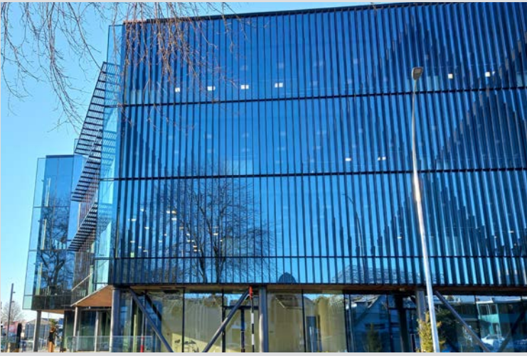
Project Hauata offices for ACC, Hamilton - PW1000 with integrated vertical box louvre fins, and horizontal solar shade louvres.
