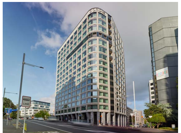
Cordis Hotel, Auckland - PW1000 Unitised Structurally Glazed Curtainwall
