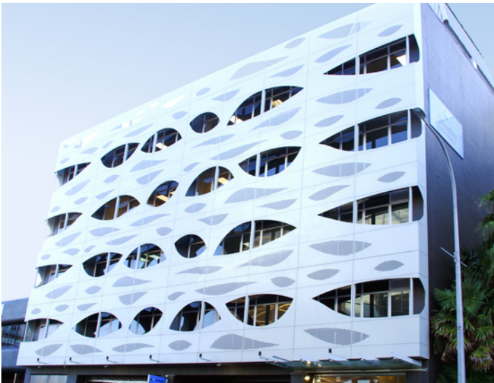
15 Huron St, Auckland - laser cut aluminium cladding installed with ENCLAD™ EN05-FF Support System.
