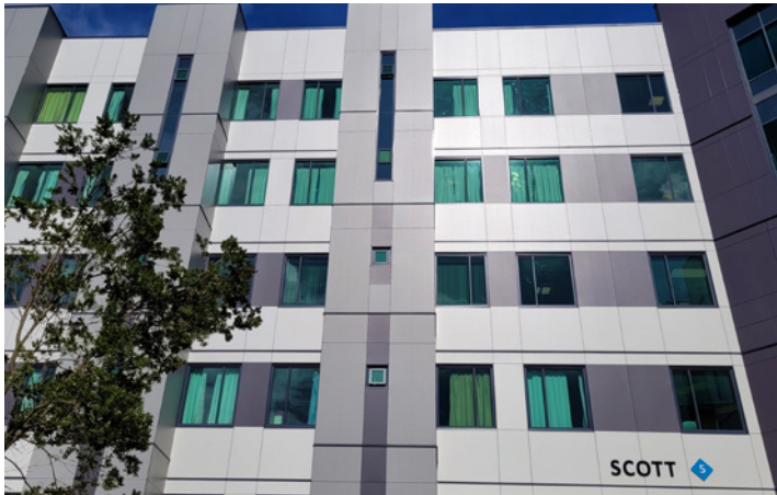
Middlemore Hospital, recladding of Scott building, Auckland - FUNDERMAX high pressure laminate installed with ENCLAD™ EN01 Support System.
