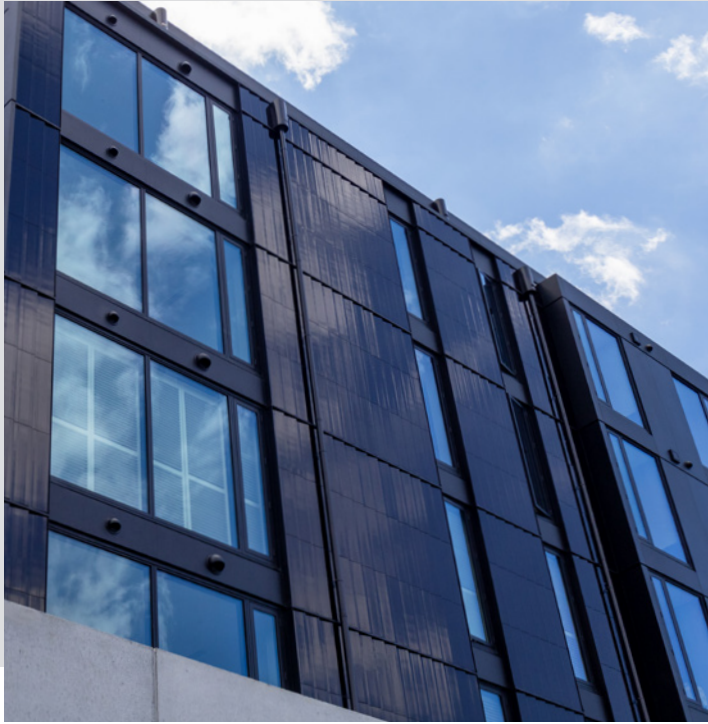
One St Stephens, Auckland - black Terracotta tile cladding vertically installed with ENCLAD™ EN03 Rainscreen Support System.
