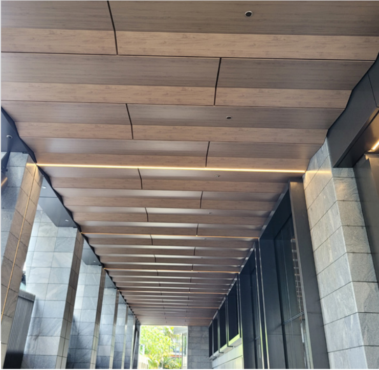
Cordis Hotel, Auckland - sublimated woodgrain aluminium soffits installed with ENCLAD™ EN01 Support System
