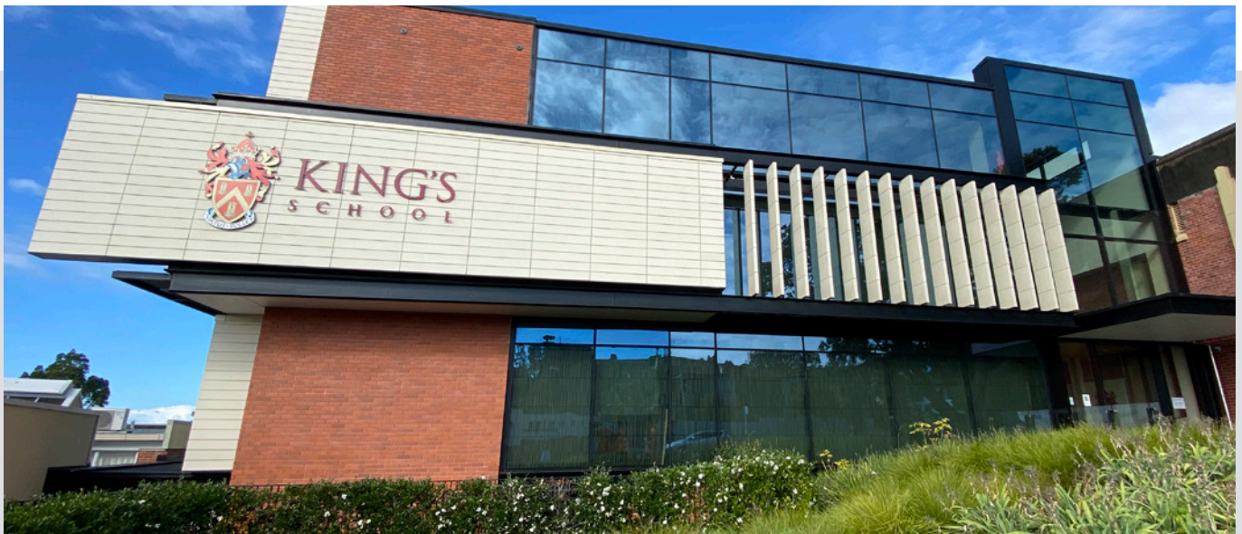
King's School, Auckland - Terracotta tiles horizontally installed with ENCLAD™ ENO2 Rainscreen Support System.
