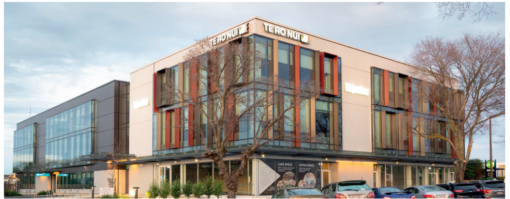
Te Ao Nui (IL4) Building, Palmerston North - RS1000 Cladding System hooked-on folded sheet metal and aluminium plank cladding, vertically and horizontally fixed.
