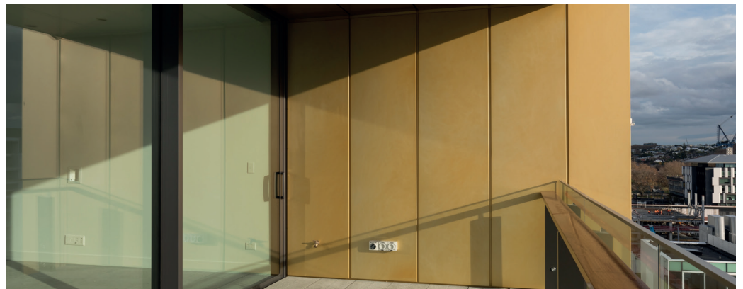
Halsey St, Auckland - RS1000 Cladding System
