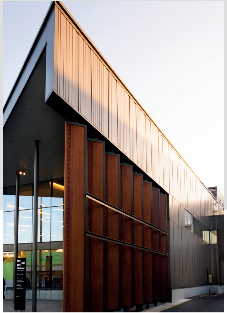
Johnsonville Library - RS1000 Cladding System incorporating powdercoated aluminium vertically and horizontally fixed
