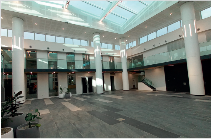
Toyota, Palmerston North - WS1000 system curved aluminium column claddings
