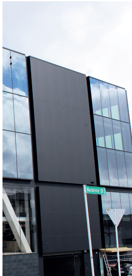
Giltrap Prestige Building, Auckland - WS1000
