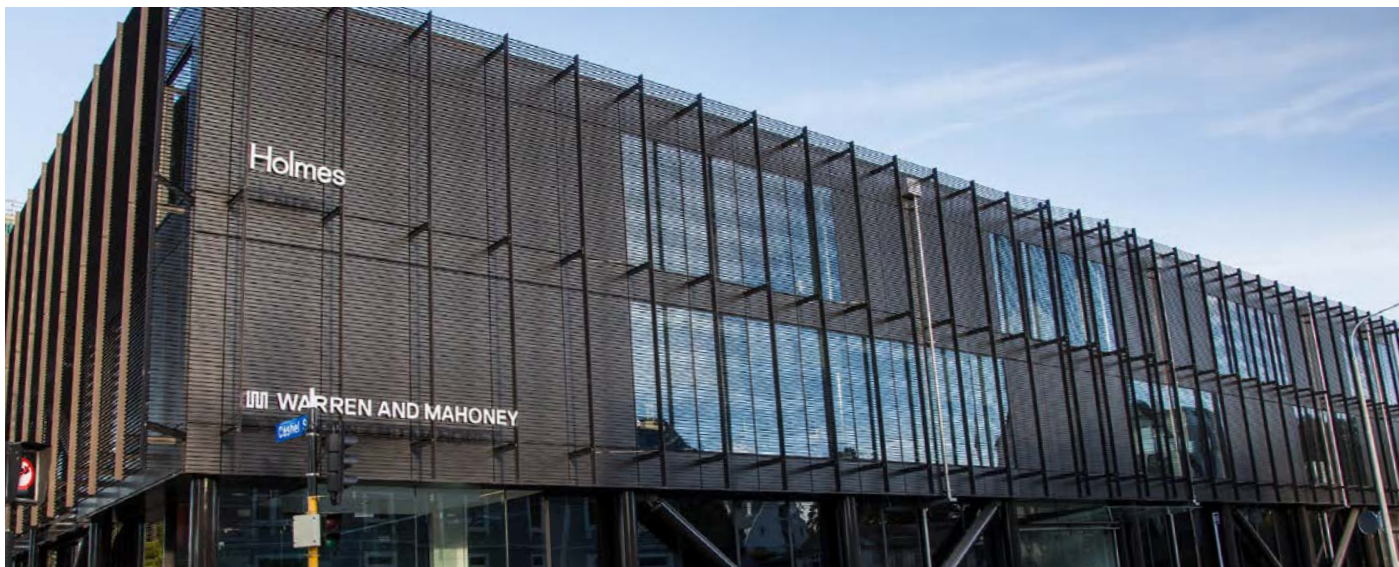
Warren & Mahoney offices in Christchurch - Shadegrade™ installed as solar shading to exterior facade.
