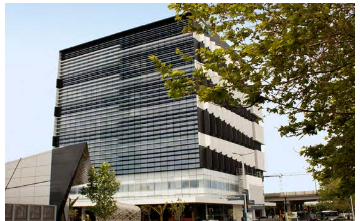
Sylvia Park Office Tower, Auckland - Horizontal and vertical solar shade elements.
