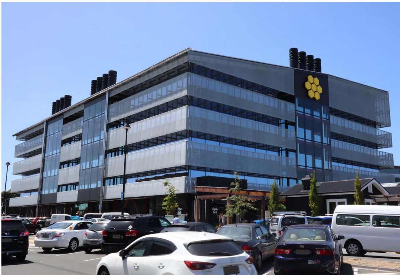
Smales Farm B-Hive, Auckland - Web grate solar shading screens.
