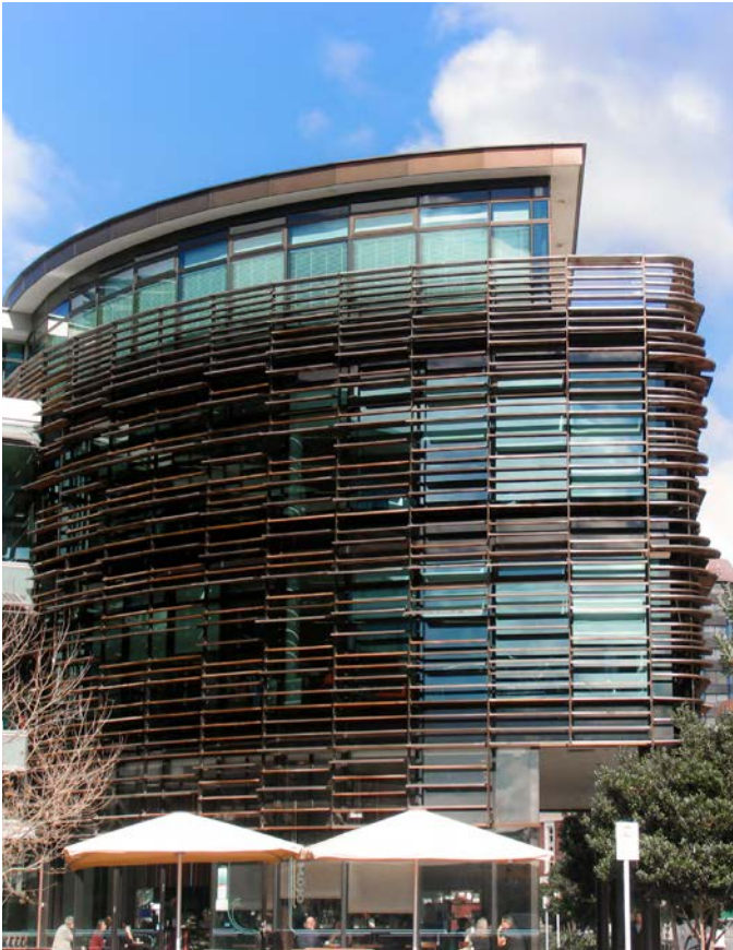
Meridian Energy Site 7, Wellington - Timber louvres integrated into curtainwall.
