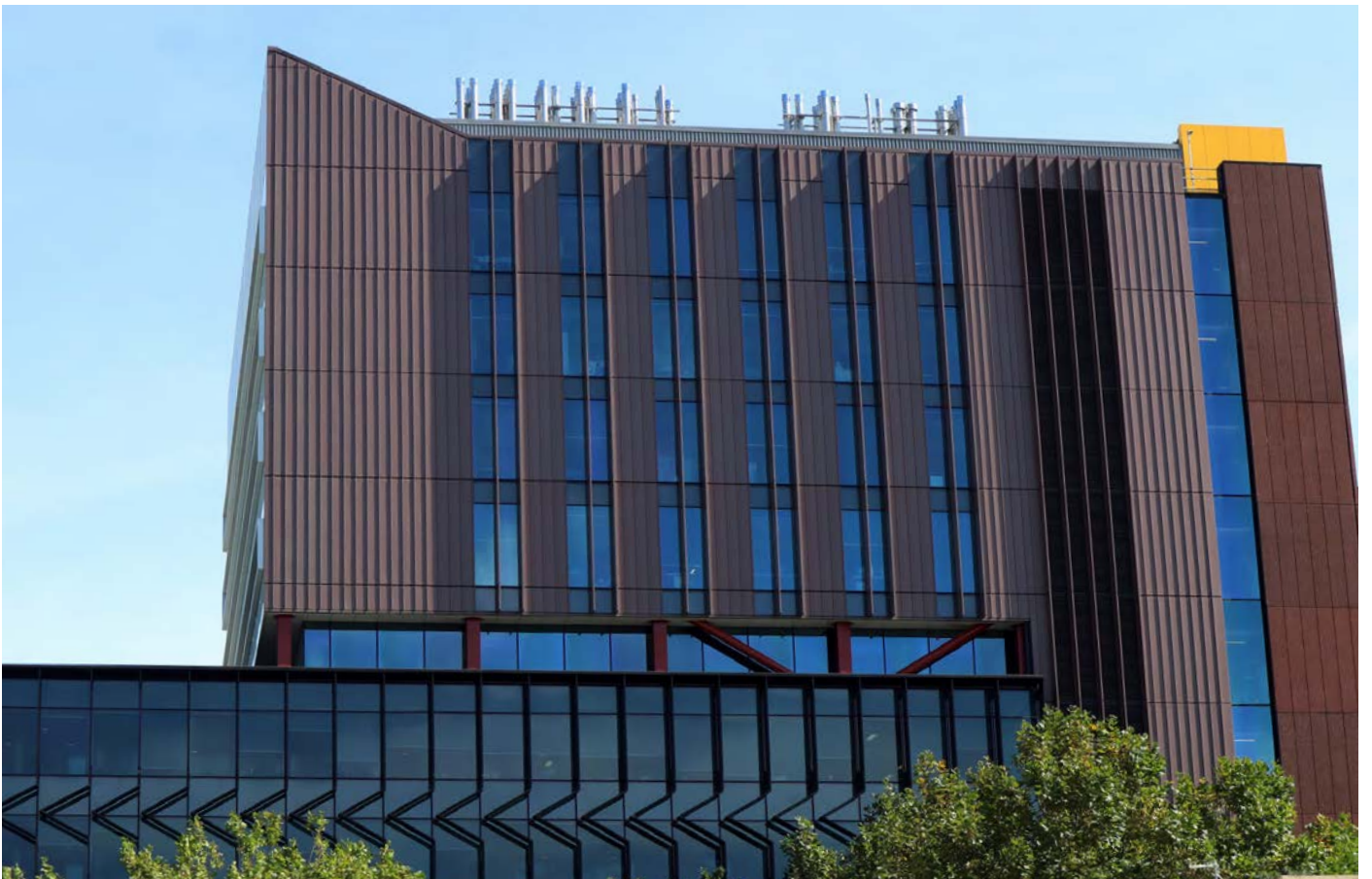
University of Auckland, School of Science 302 - Large chevron feature elements integrated into Thermosash PW1000 unitised curtainwall, and zinc clad vertical fins.
