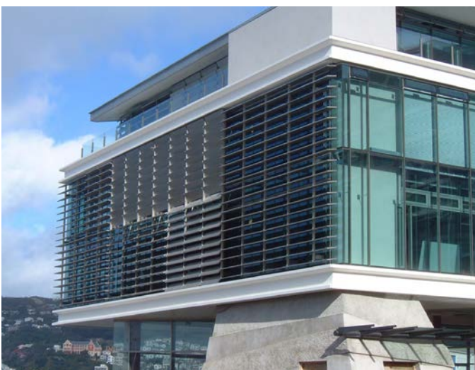
Meridian Energy Site 7, Wellington - Automatic window and louvre actuators, providing passive heating and cooling of the building.
