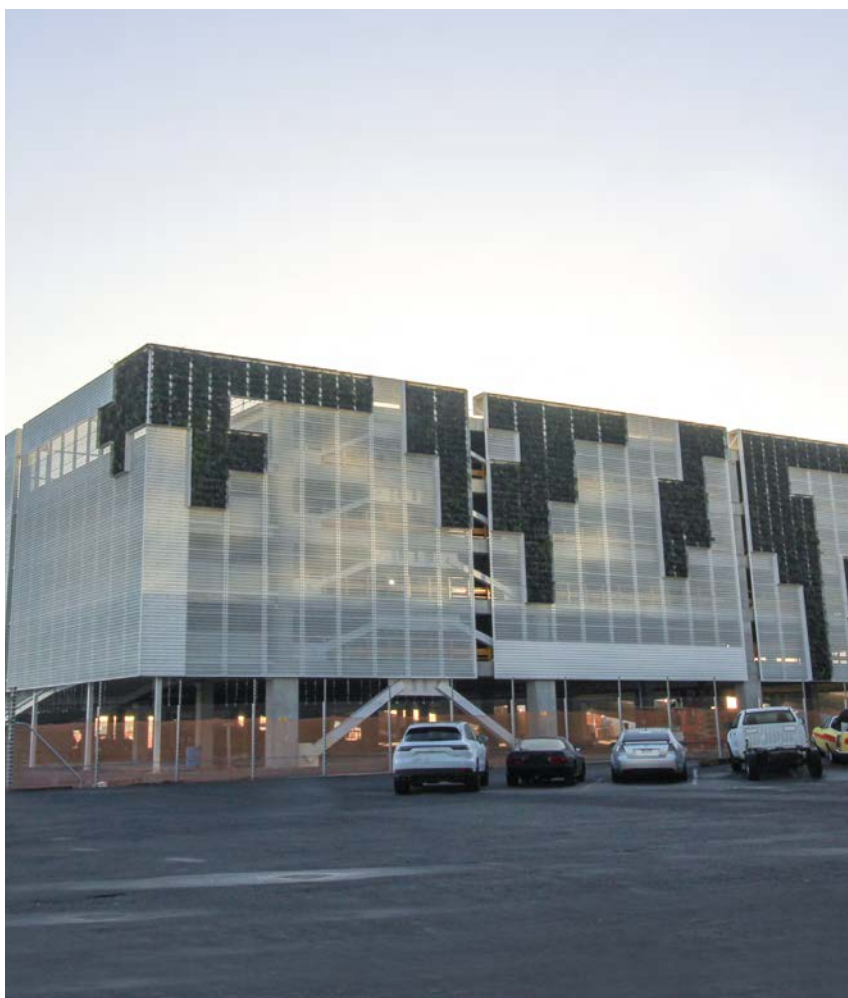
Blesdisloe Wharf Carpark, Auckland - Unitised perforated sheet metal incorporating an integrated green wall.
