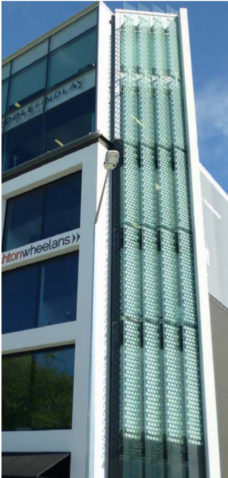
83 Victoria street, Christchurch - Frit glass louvres levels 1-5 of the 6 storey building.
