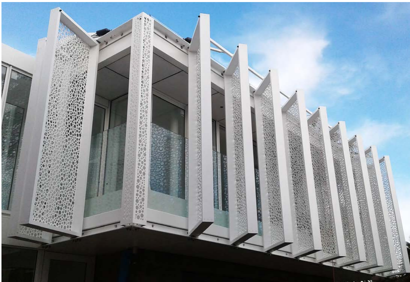
Paritai Drive, Auckland - Perforated solar shade vertical fin screens with actuators.
