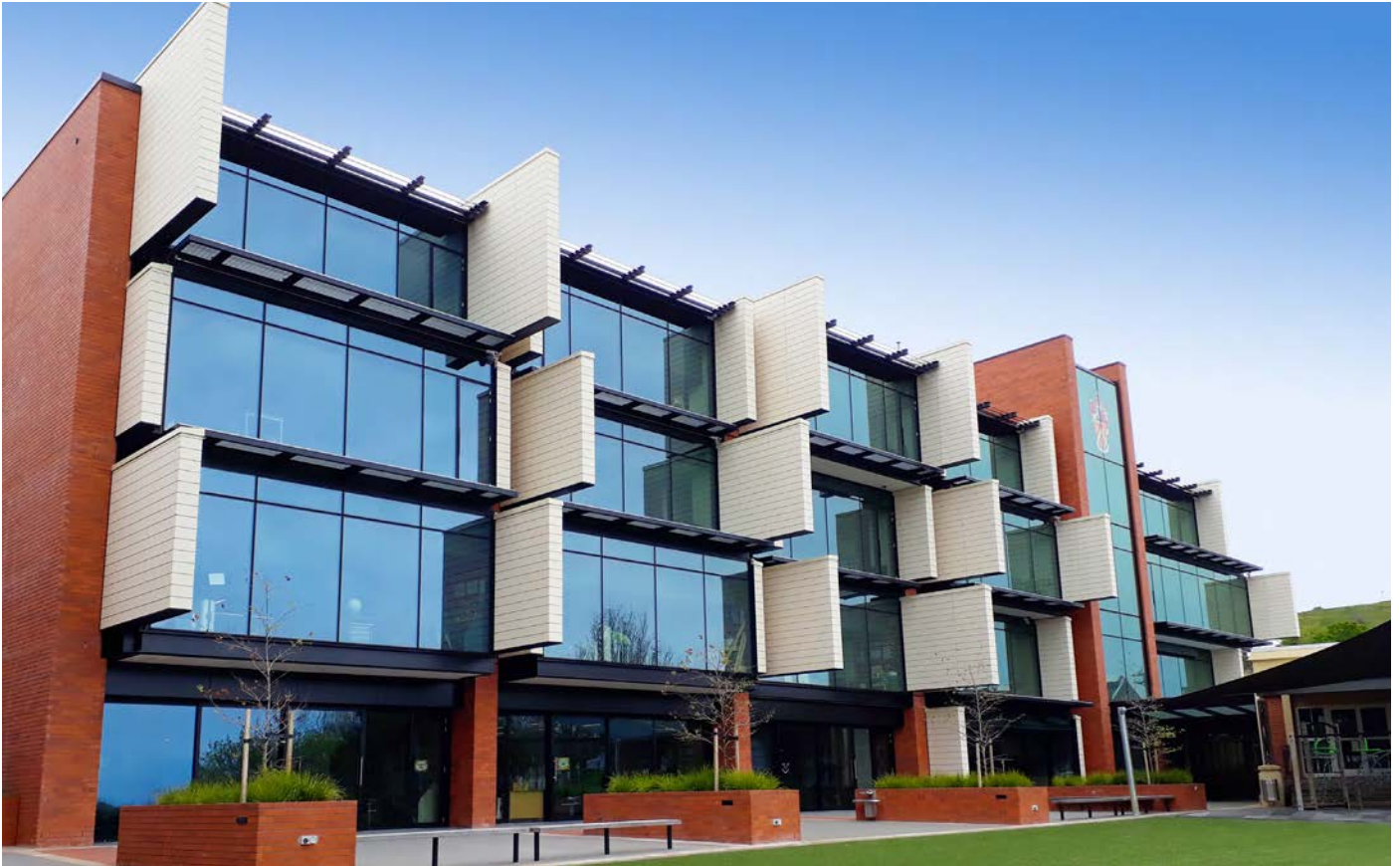
Hanna Building, King's School, Auckland - Terracotta tile solar shade vertical wings.
