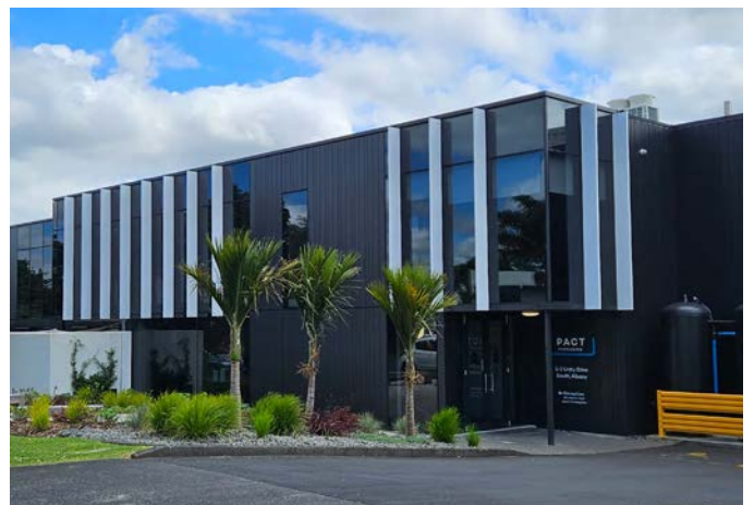
1-3 Unity Drive, Albany, Auckland - Fixed vertical solar shade fins integrated into Thermosash PW1000 unitised curtainwall.
