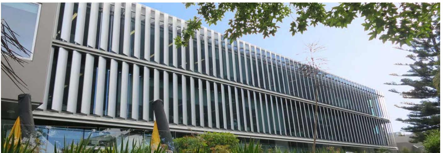
Napier Street GHD building, Auckland -Aluminium solar shade fins
