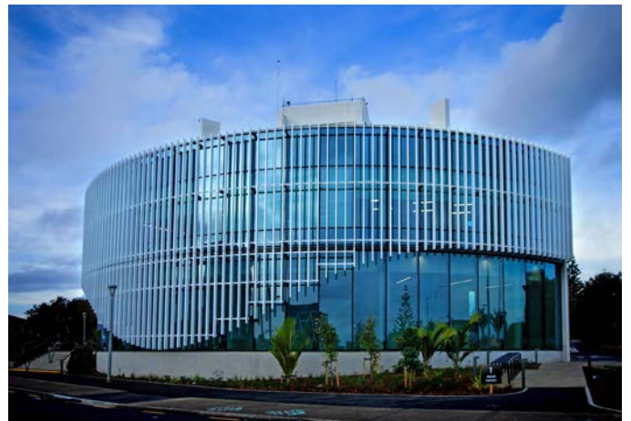
Manukau Hub, Auckland - Vertical solar shade fins integrated into Thermosash PW1000 unitised curtainwall.
