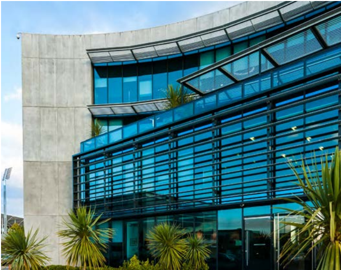
Showplace, Christchurch - PW400 Unitised Curtainwall with integrated horizontal solar shade louvres.
