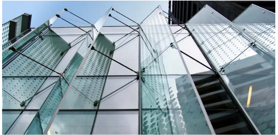
Lambton Square Plaza, Wellington - Frit glass louvres with actuators
