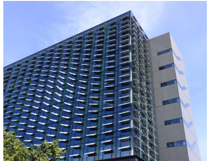
University of Auckland Engineering 405 - Fixed external sunshades integrated into Thermosash PW1000 double glazed curtainwall.
