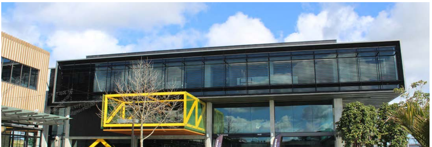
Westgate Library - Horizontal solar shade louvres
