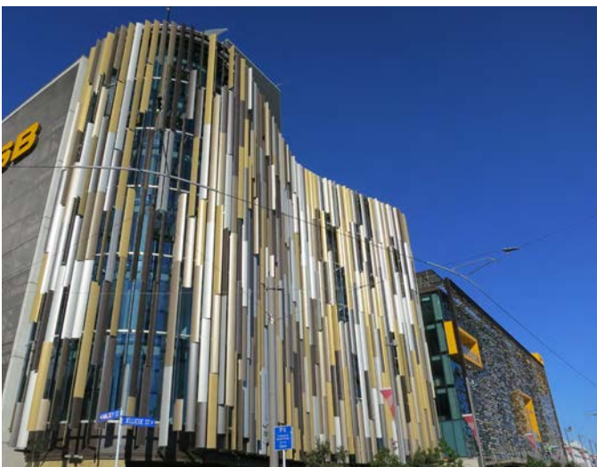
ASB North Wharf, Auckland - Vertical solar shade fins suspended off the curtainwall face.
