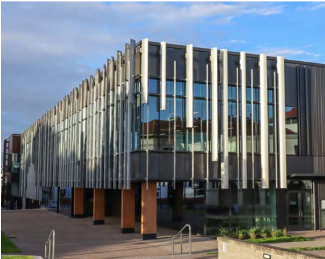
Massey University Innovation Complex - Extruded aluminium solar shading integrated into facade.
