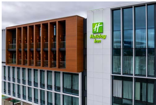
Holiday Inn Remarkables Park, Queenstown - Vertical and Horizontal solar shade elements.
