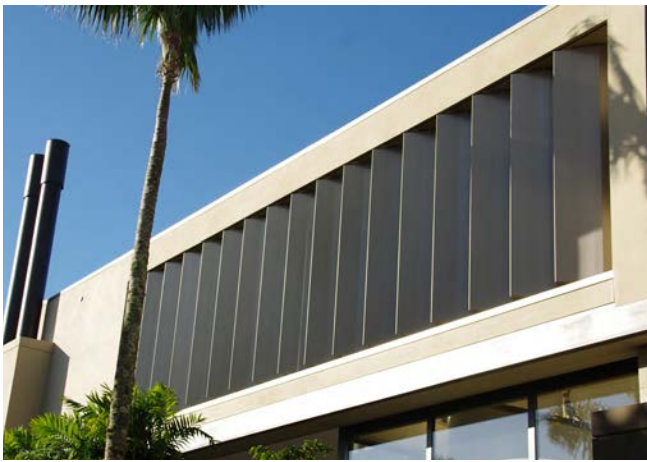
Private residence, Mission Bay, Auckland - Fully automated solar shade louvres
