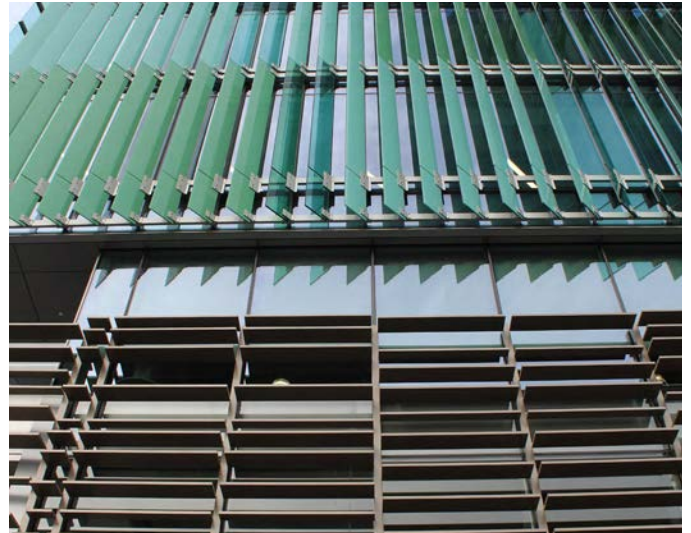
Fonterra Building, Fanshawe Street, Auckland - Vertical and horizontal solar shade louvres
