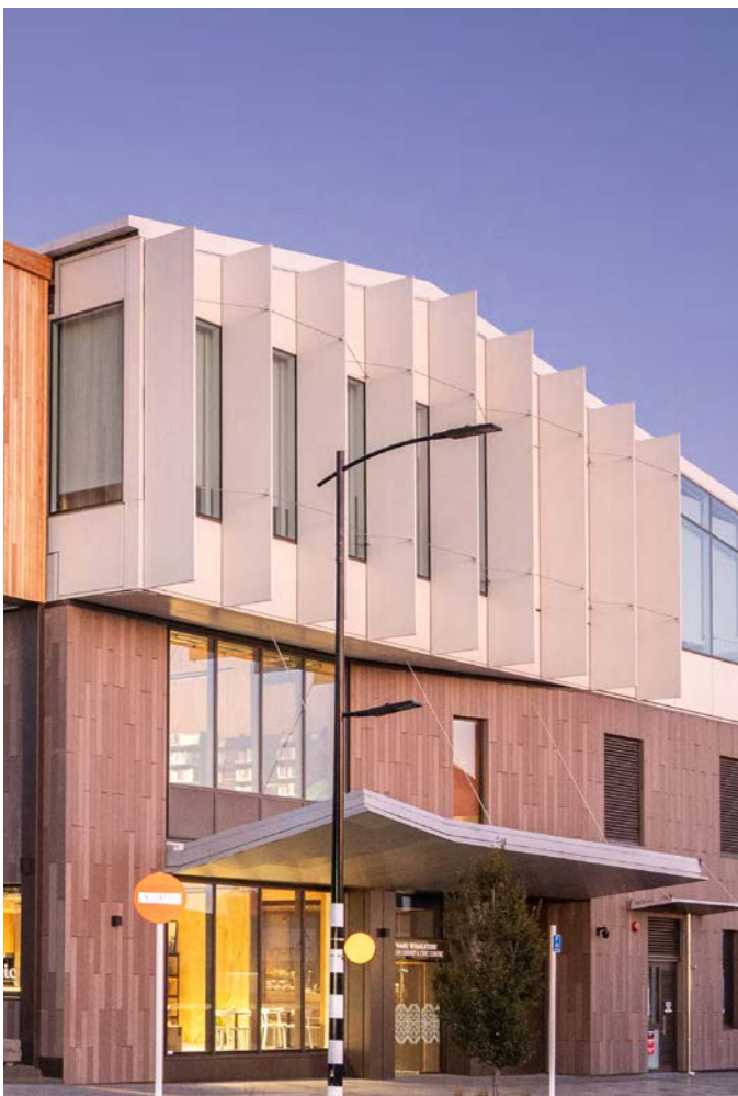
Ashburton Civic Centre & Library, Te Whare Whaktere - Thermosash PW1000 unitised curtainwall integrated with vertical solar shading fins with actuators
