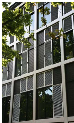
University of Auckland, Thomas Building - Integrated sunscreen
