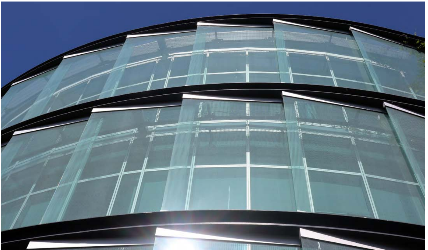
University of Auckland, Thomas Building - Frit glass structural external twin skin louvres.
