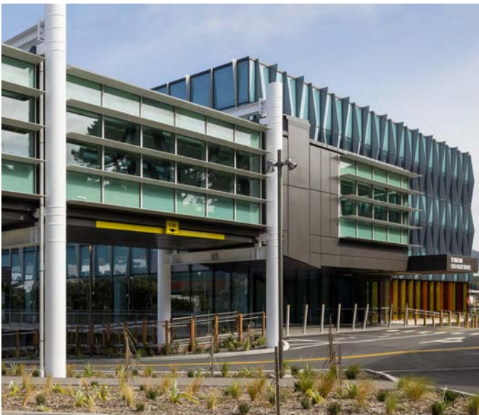
Wellington Regional Children's Hospital - Horizontal and vertical solar shading integrated into PW1000 unitised curtainwall.
