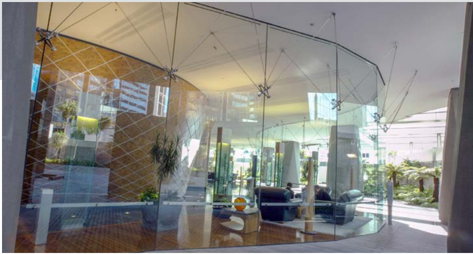
Royal Sun Alliance, Auckland - light weight structural tension cables and support fixtures on straight and angled channel glazing, provides minimal intrusive wind bracing
