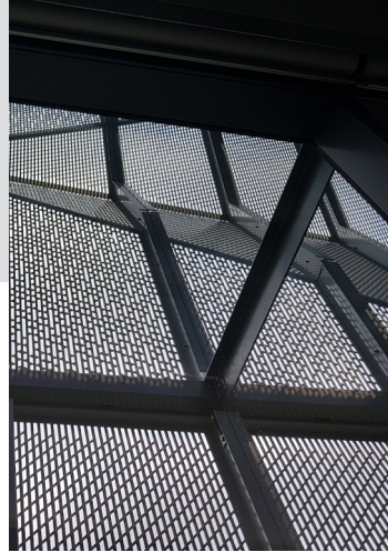
UOC - Rutherford Regional Science & Innovation Centre - 'X Chromosome' perforated architectural metal folding integrated into unitised curtainwall
