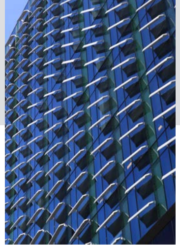
UOA Engineering 405 - custom sunshade elements integrated into unitised curtainwall
