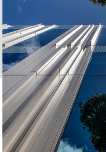
University of Auckland, B201 - unitised aluminium plank
