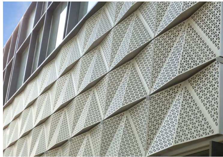
Bnz Cashel stage 1 - perforated and folded sheet metal installed as car park screening
