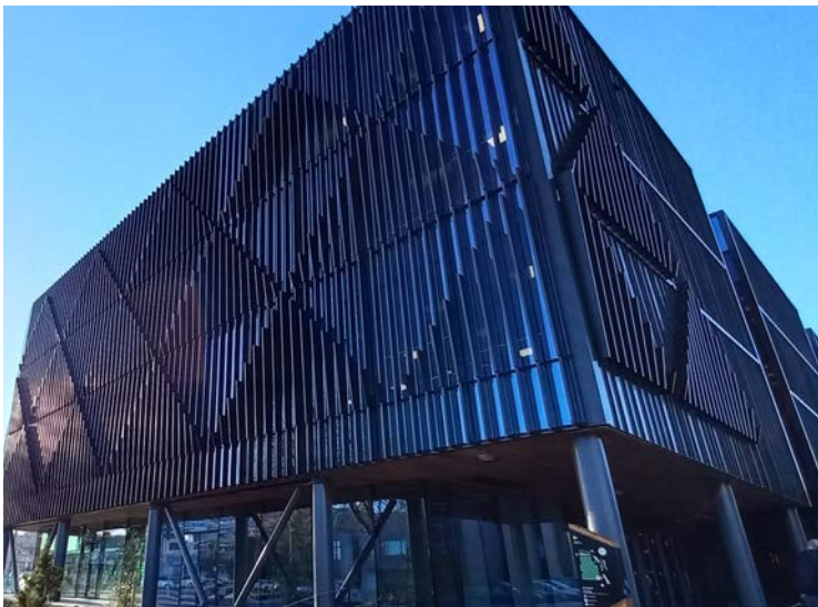
Project Hauata, ACC, Hamilton - vertical box louver fins integrated into Thermosash PW1000 unitised curtainwall
