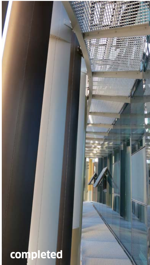
Shadetread™ external facade service access behind vertical sunshade elements and integrated into PW1000 Unitised Curtainwall - ASB North Wharf, Auckland
