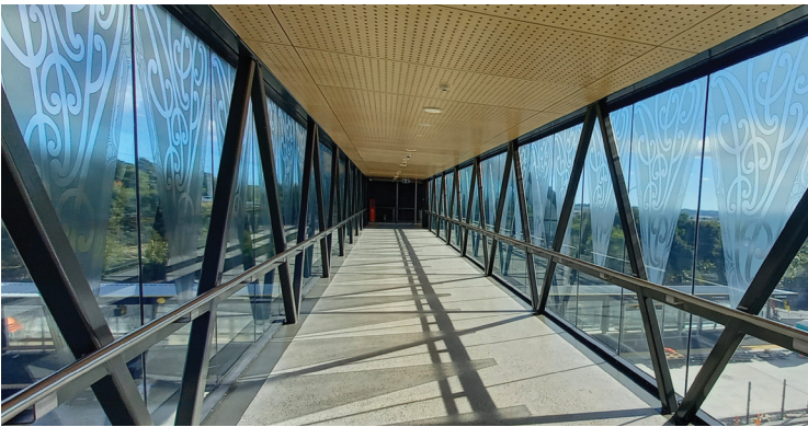
Constellation Bus Station, Auckland - channel glazed pedestrian overpass
