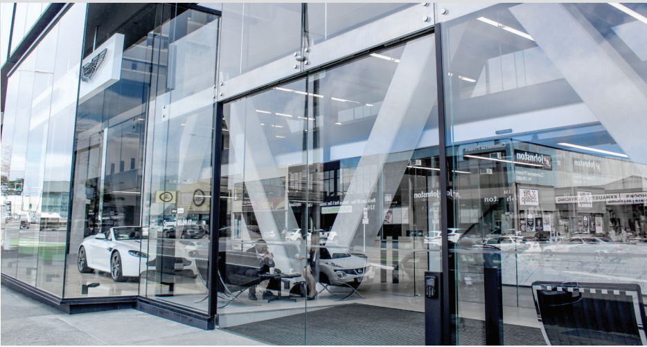
Giltrap Prestige, Auckland - channel glazed showroom with integrated glass fins and framed glass auto doors
