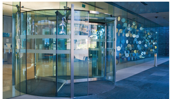
Lumley Tower, Auckland - channel glazed entrance incorporating revolving door
