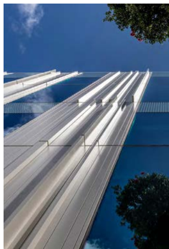
University of Auckland B201 - unitised aluminium planking integrated.
