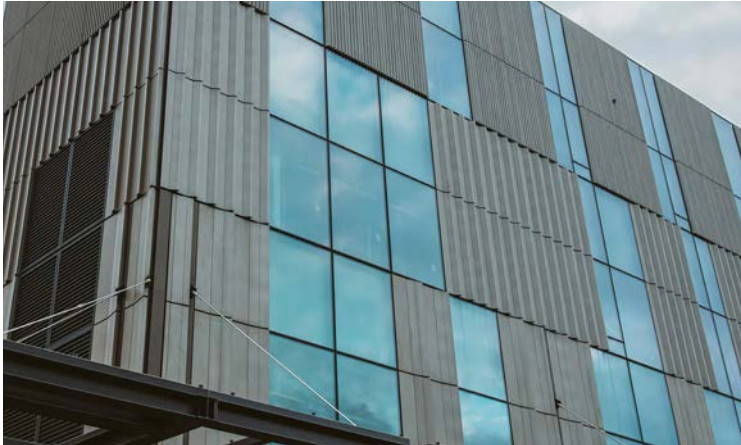
Taranaki Base Hospital Extension - unitised aluminium planking integrated into PW1000 High Performance Unitised Curtainwall.
