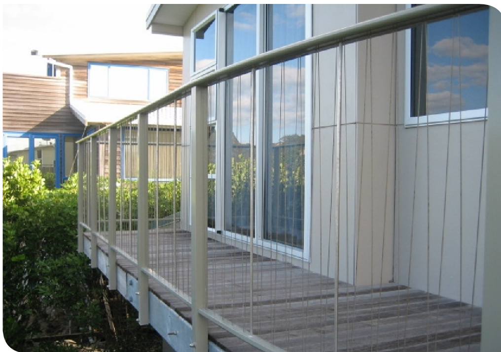
Figure 4.13 Sloping wires changing direction within the rails
