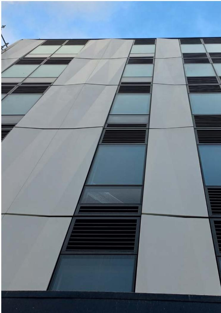
1 Enfield Apartments - architectural aluminium pressings integrated into curtainwall.
