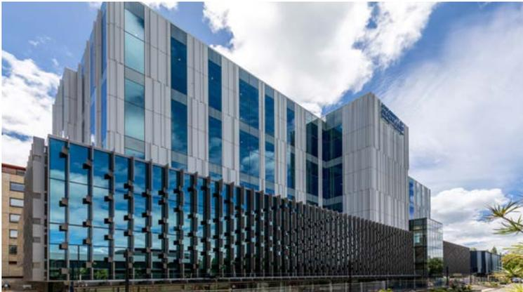
University of Auckland B201 - unitised aluminium planking integrated with PW1000 HP Unitised Curtainwall delivers an energy efficient envelope.
