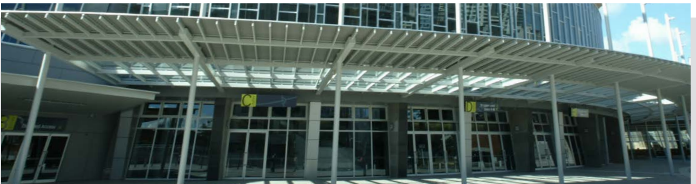
Spark Arena (formerly Vector Arena), Auckland - Thermosash Alpha Glazing System installed as a large glazed canopy.
