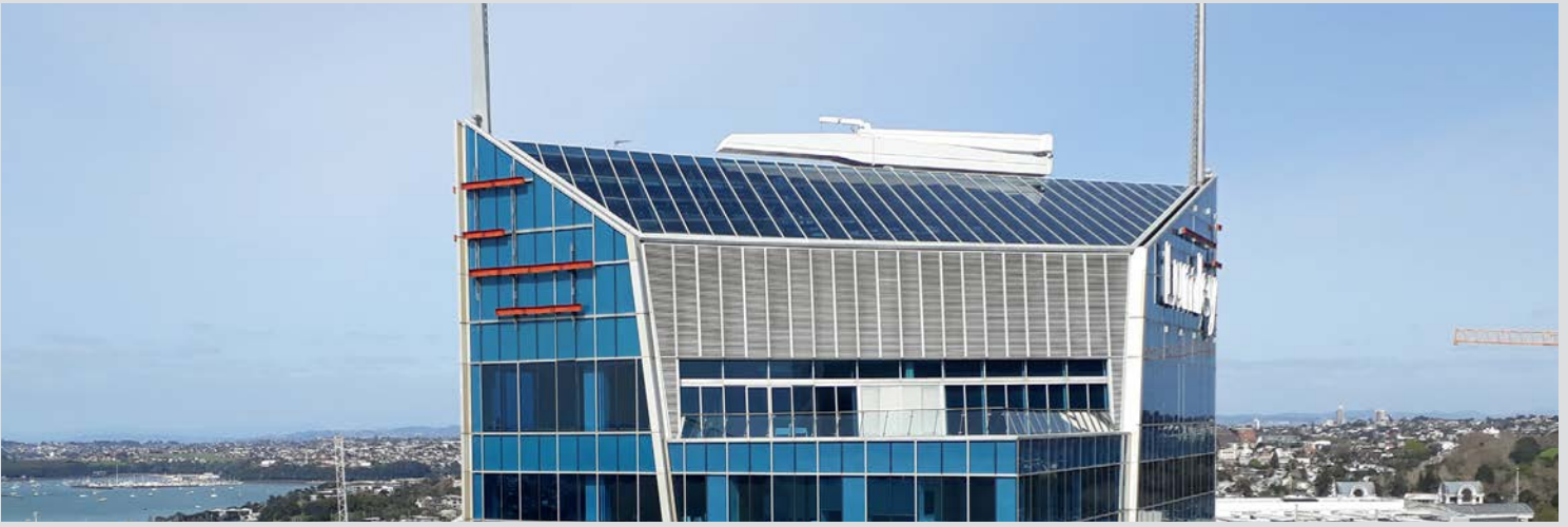
Lumley Tower, Auckland CBD - Thermosash Alpha Glazing System installed to the entire roof
