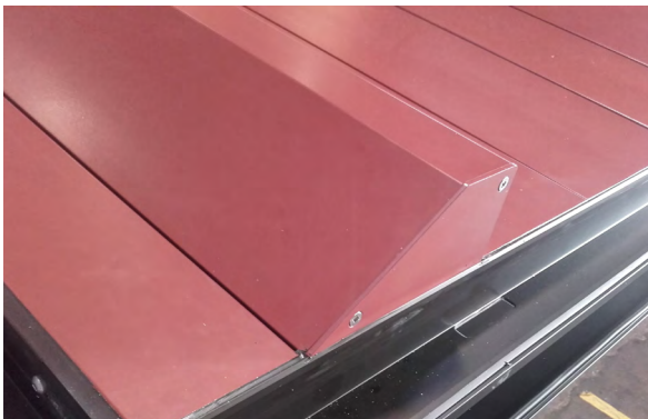
AUT M1 Mana Hauora Building - unitised aluminium planking provided a lightweight alternative to terracotta due to the floor spans on this project.
