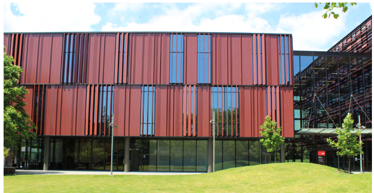
AUT M1 Mana Hauora Building - unitised aluminium planking provided a lightweight alternative to terracotta due to the floor spans on this project.
