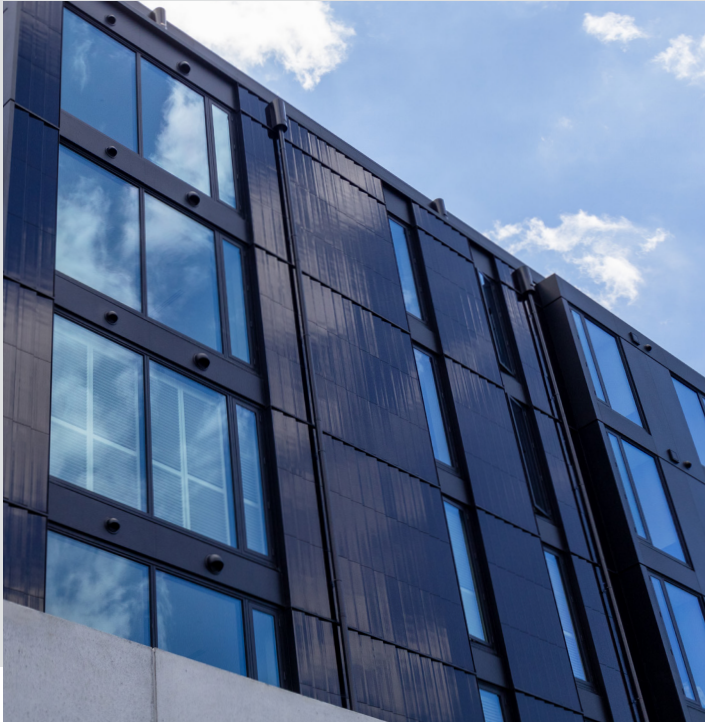
One St Stephens, Auckland - black Terracotta tile cladding vertically installed with ENCLAD™ EN03 Rainscreen Support System.
