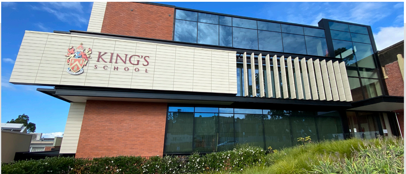
King's School, Auckland - Terracotta tiles horizontally installed with ENCLAD™ EN02 Rainscreen Support System.
