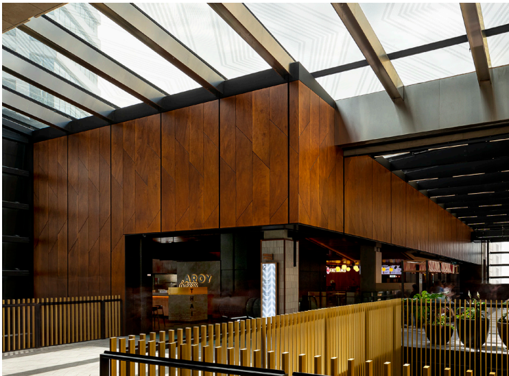
Commercial Bay, Auckland - interior PRODEMA High Pressure Laminate installed with ENCLAD™ EN01 Support System.
