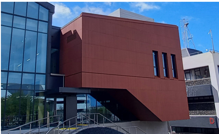
Otago Polytechnic Trades Training Building, Dunedin - Terracotta tile cladding vertically installed with ENCLAD™ EN03 Rainscreen Support System.
