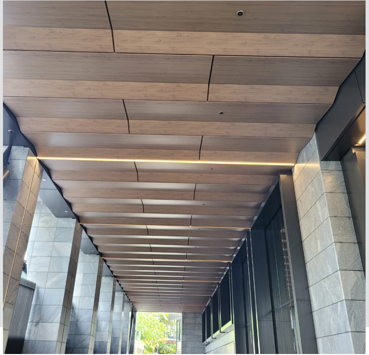
Cordis Hotel, Auckland - sublimated woodgrain aluminium soffits installed with ENCLAD™ EN01 Support System
