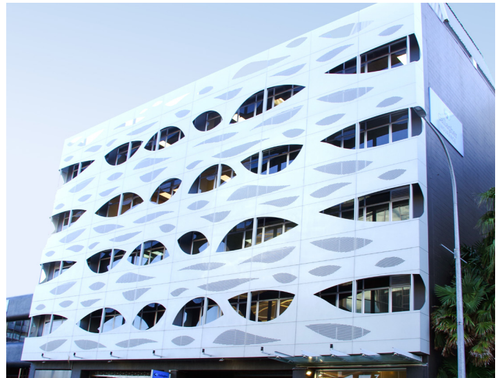
15 Huron St, Auckland - laser cut aluminium cladding installed with ENCLAD™ EN05-FF Support System.
