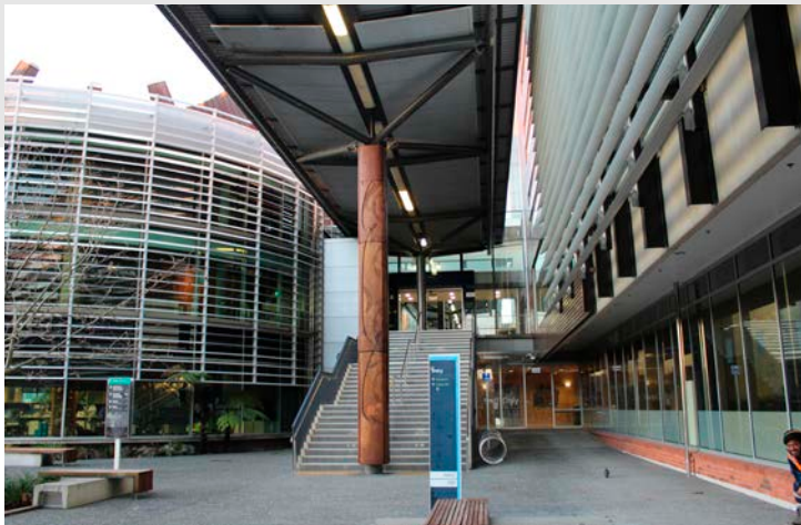
Waitakere Civic Centre, Auckland - PW400 Unitised Curtainwall installed as secondary glazing to Civic building and primary curtainwall to Admin block.
