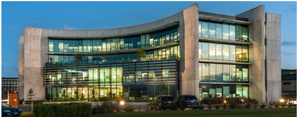
Showplace, Christchurch - PW400 Unitised Curtainwall with integrated solar shading
