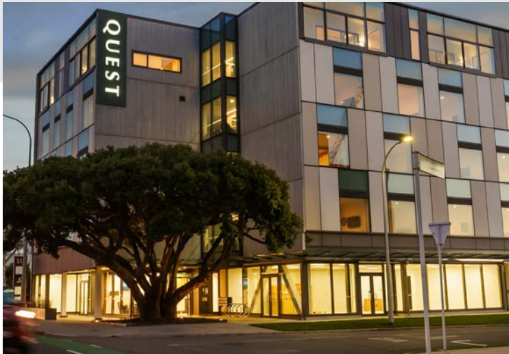
Quest Hotel, Takapuna - PW400 Unitised Curtainwall Suite to the ground floor
