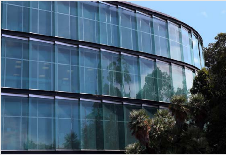
UOA Thomas Building - PW400 Unitised double glazed curtainwall with external skin structural glass louvres
