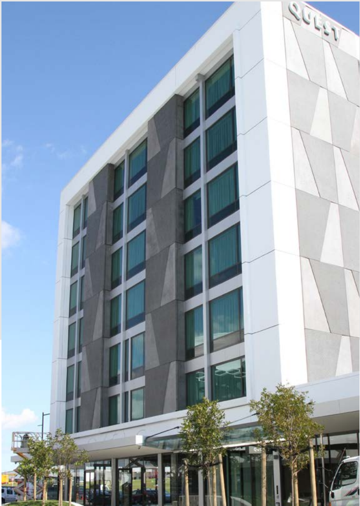
The Crossing, Quest Hotel, Auckland - PW400 Unitised Curtainwall
