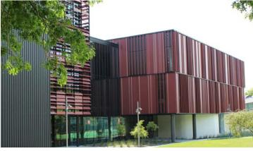
AUT M1 Mana Hauora Building - unitised aluminium planking provided a lightweight alternative to terracotta due to the floor spans on this project.
