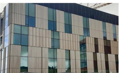
Taranaki Base Hospital Extension - unitised aluminium planking integrated into PW1000 Factory extruded and folded Aluminium planking unitised panels High Performance Unitised Curtainwall.
