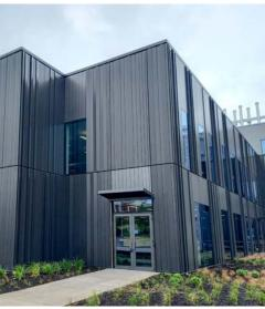
Massey Innovation Complex, Auckland - unitised extruded aluminium plank integrated with PW1000 aluminium plank vertical cladding. HP Unitised Curtainwall.
