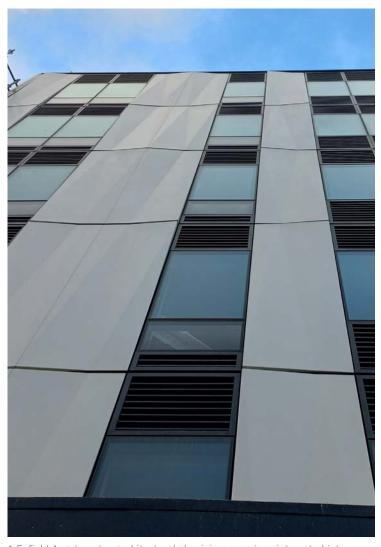
$1 \ {\sf Enfield Apartments} \ {\sf - architectural \ aluminium \ pressings \ integrated \ into \ curtainwall.}$
