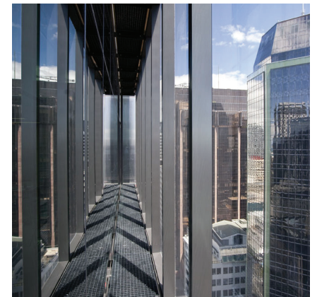
Shadetread™ access walkway in twin-skin curtainwall system - Deloitte, Auckland
