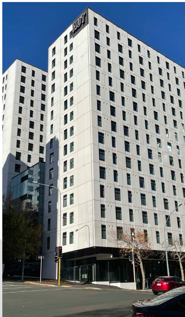
AUT Student Accommodation DELTA SUITE WINDOWS
