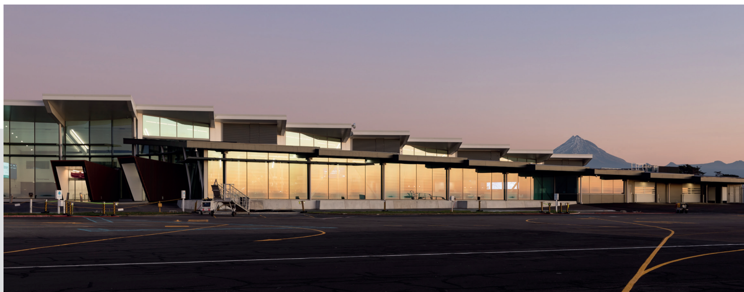
New Plymouth Airport - PW1000 Unitised Curtainwall with a complex grid and structural frame incorporating large panes of glass.
